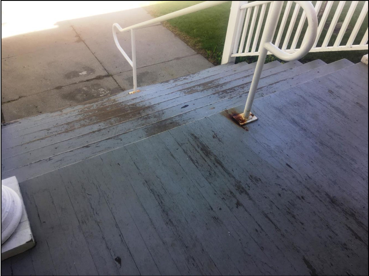
Figure 3. Deck view of Library stairs.
