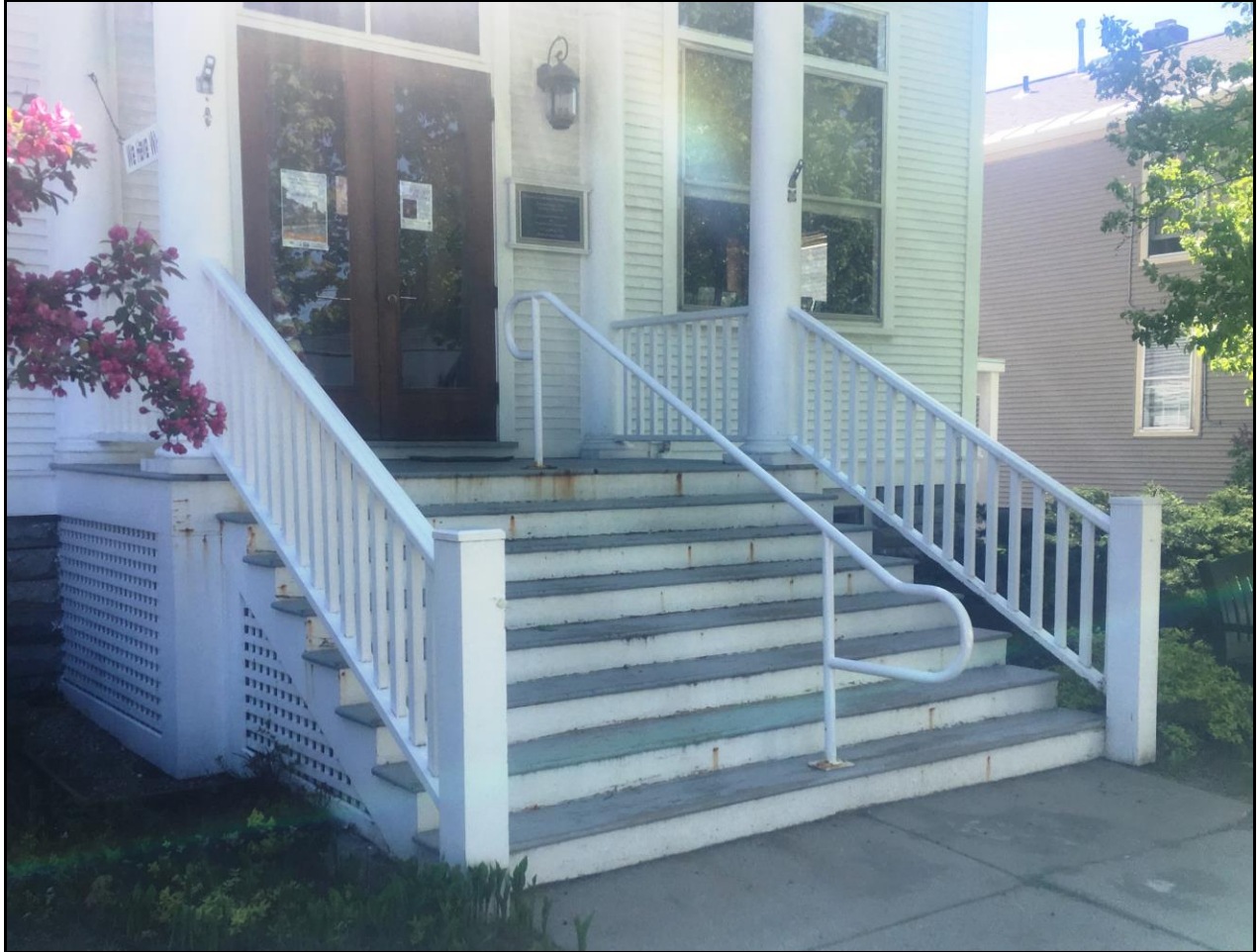
Figure 1. Lawrence Lane view of the stairs.
