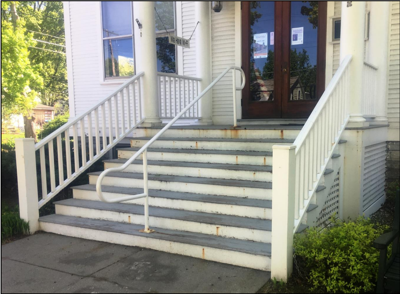
Figure 2. North Street view of Library stairs.
