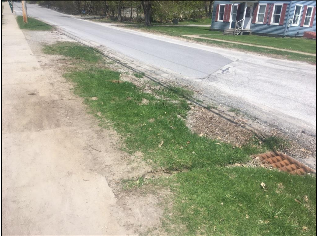
Figure 9. Mountain Street sidewalk and drainage issue. The sidewalk will need to be elevated to eliminate the ponding. (05/09/2018).
