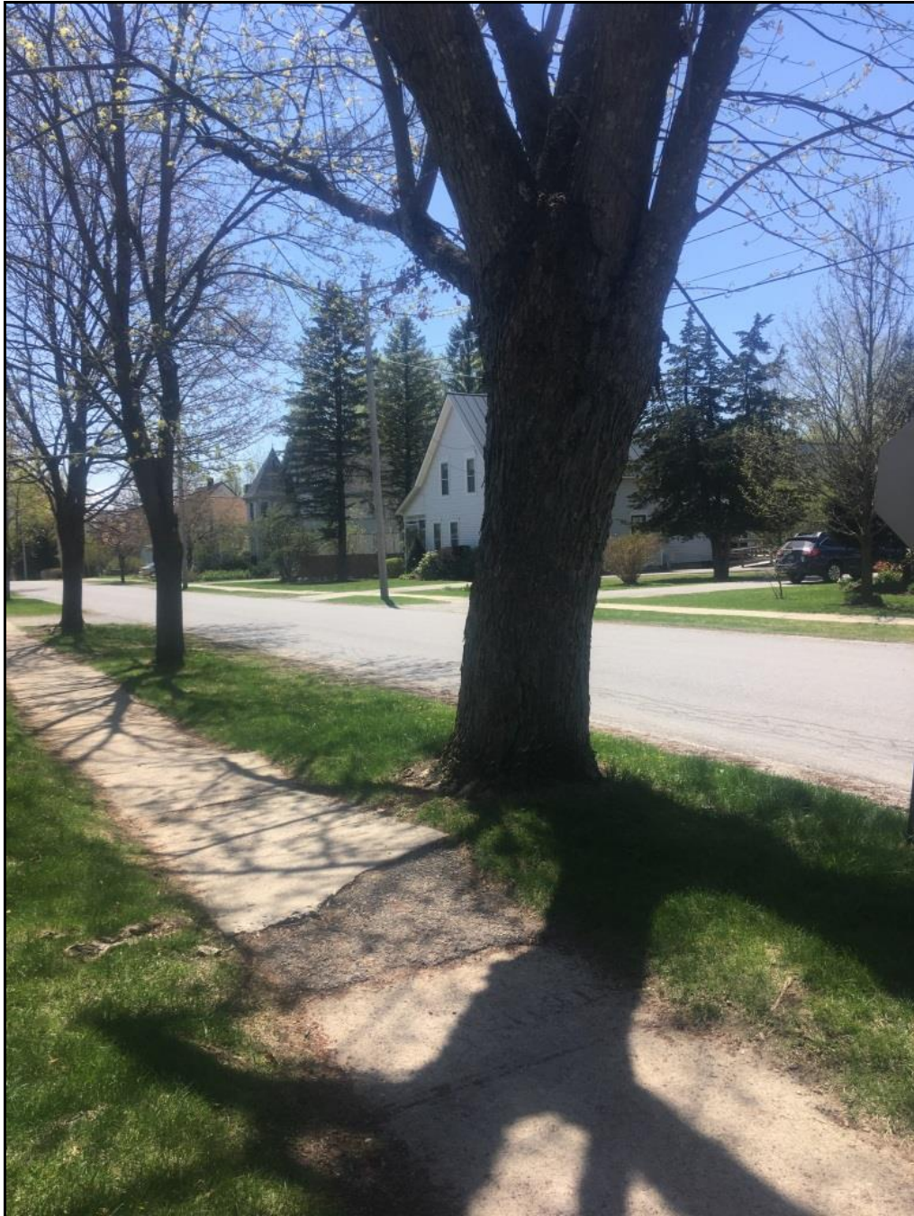
Figure 7. Maple Street sidewalk tree root damage. (05/09/2018).
