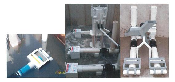
Failed siphons are readily replaced with Flouts.
