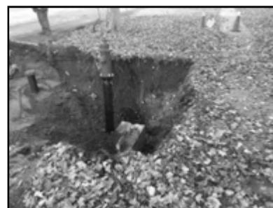
New Hydrant & Valve on West Street
