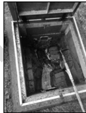
Influent Hatch After Grease Removal and Cleaning
