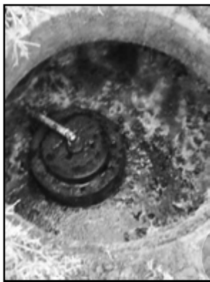
Dosing Siphons Before Cleaning
