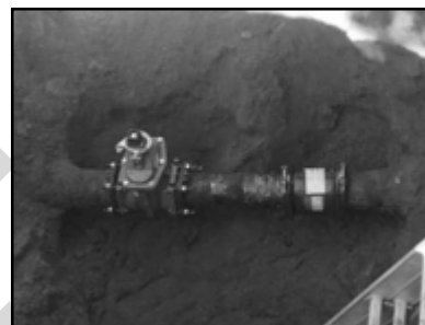
New Valve at the Corner of Pine & Taylor Replacing Old Valve
