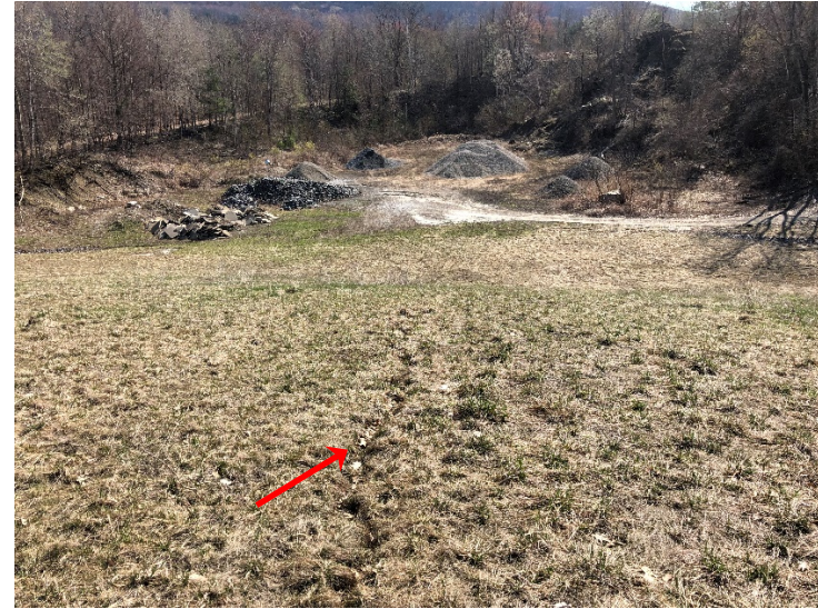
Photo #10: Erosion on northeast slope
