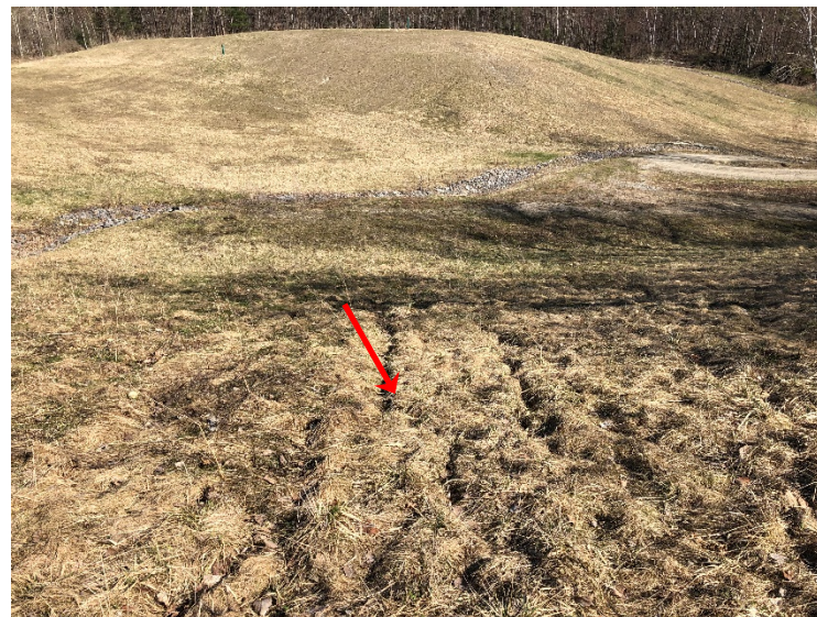
Photo #2: Closeup of eroded areas on north facing southern limit
