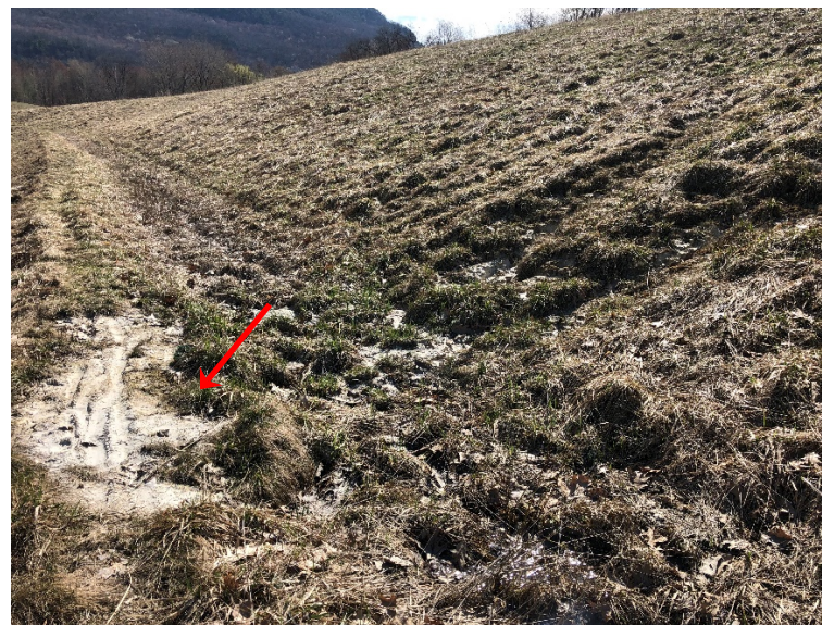
Photo #8: Closeup of erosion on north facing swale
