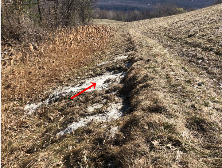
Photo #9: Erosion along drainage swale on northern limits
