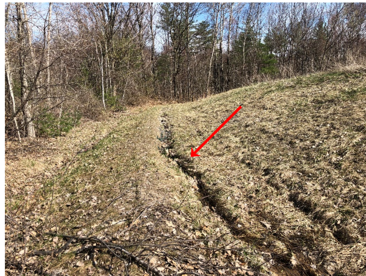
Photo #6: Eroded area on north facing drainage swale
