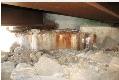
Abutment bridge seat spalling
