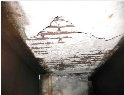
Concrete deck spalling
