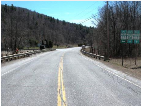
Looking South at the Bridge
