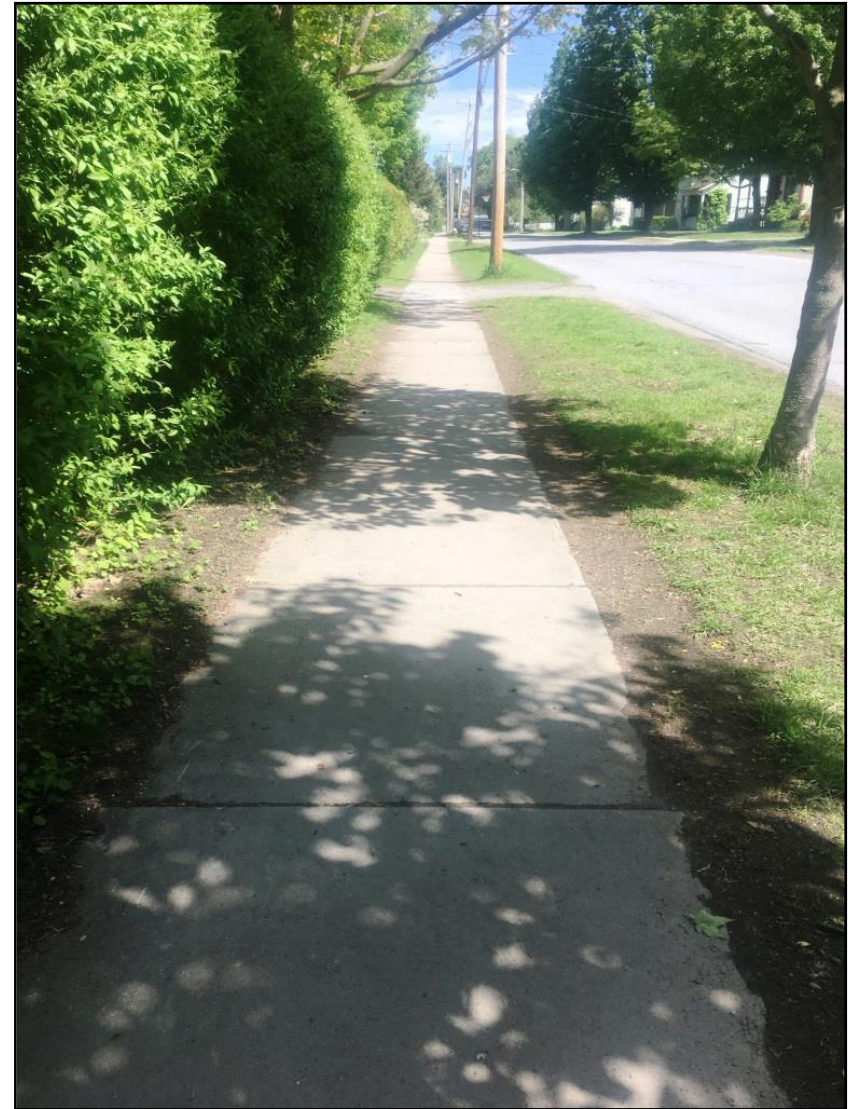
Figure 2. Mountain Street, facing north.
