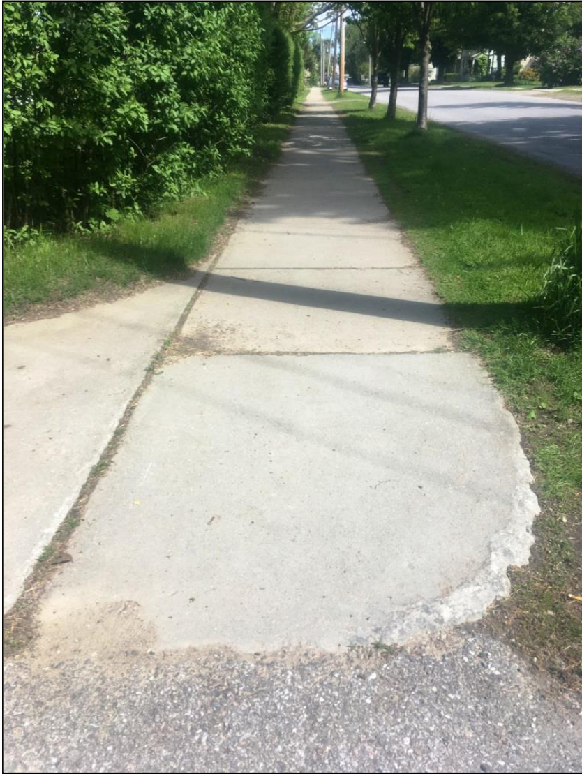
Figure 1. Mountain Street at Garfield Street.
