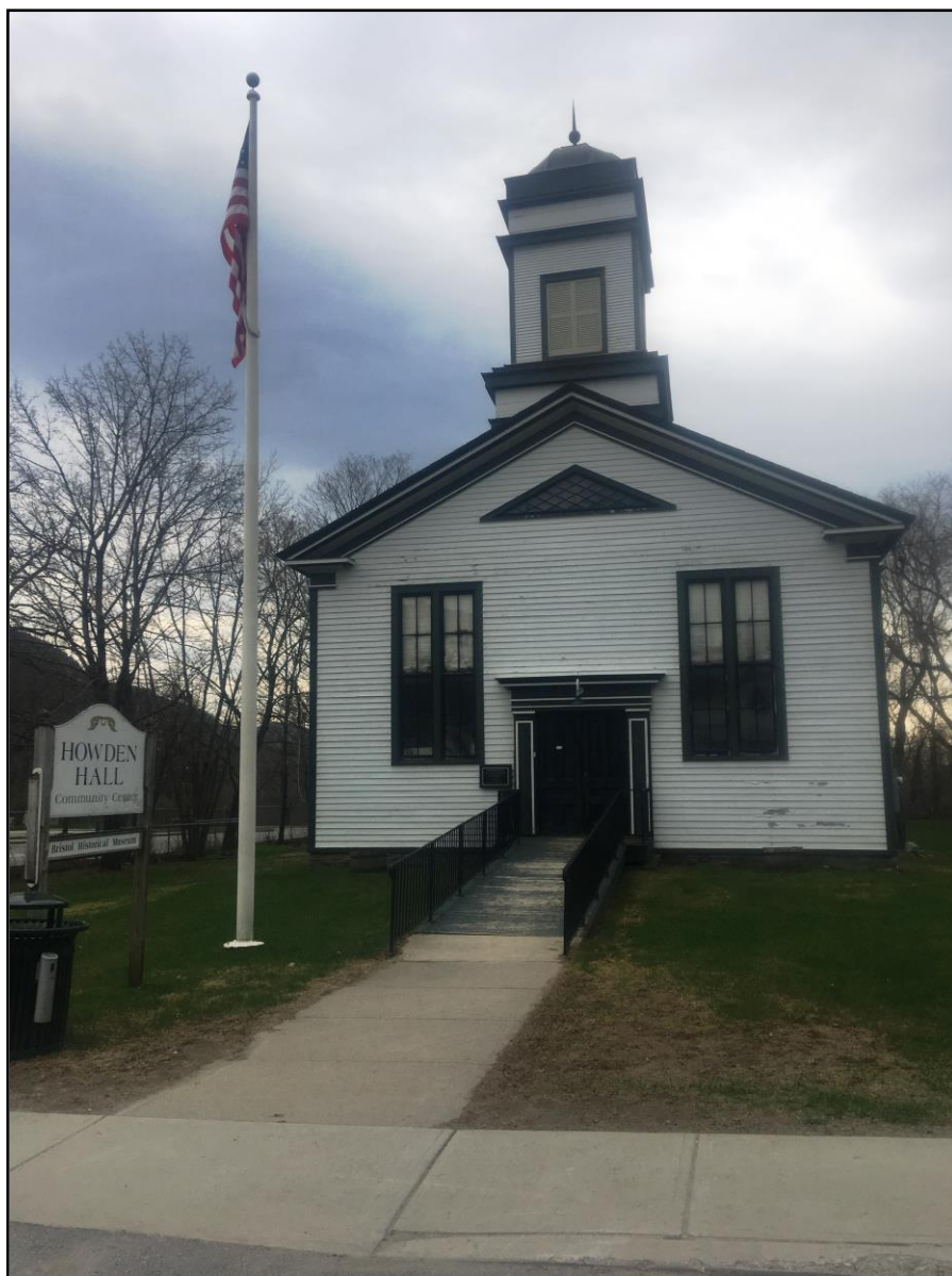
Figure 1. Howden Hall Building (front).
