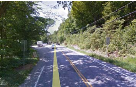
Southbound End Project MM 7.263
