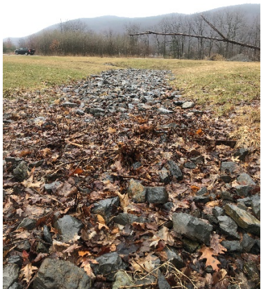
Photo #3: Main Basin Overflow Outlet
