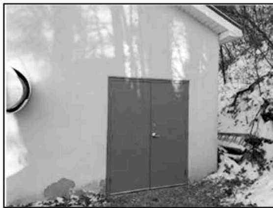
New Doors at Water Pump House
