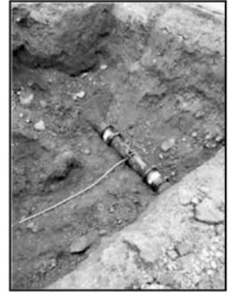
Leak Repaired with a New Service at the Post Office
