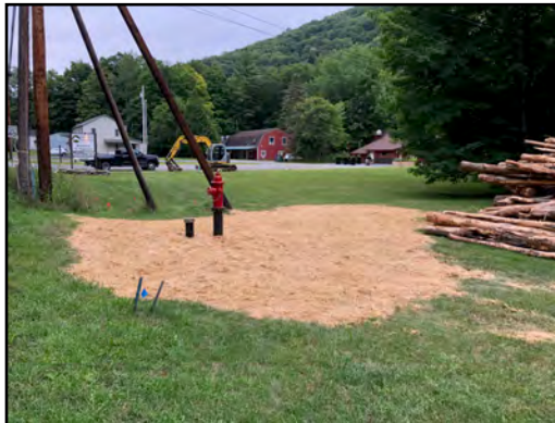
Rockydale Road – old broken hydrant. Replaced with new fully-functioning hydrant and valve
