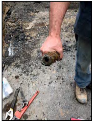
Pine Street – Replacement of leaking old galvanized service
