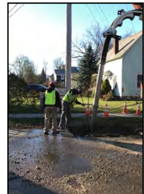
Munsill Ave - Repair to fast-leaking radial crack on 6” main
