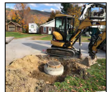
KTP Meter pit repair with added riser, waterproofing, and new meter
