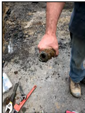
Pine Street – Replacement of leaking old galvanized service
