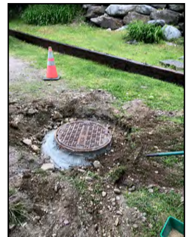
Repairs to dosing siphon manhole on South Street
