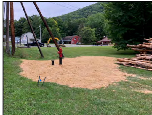
Rockydale Road – old broken hydrant. Replaced with new fully-functioning hydrant and valve
