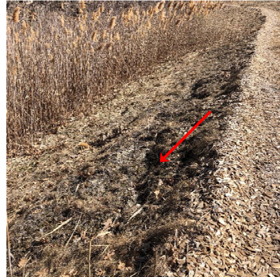
Photo #6: Eroded area on north facing drainage swale
