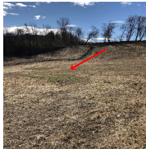
Photo #2: Erosion has been repaired in these areas on the south facing slope
