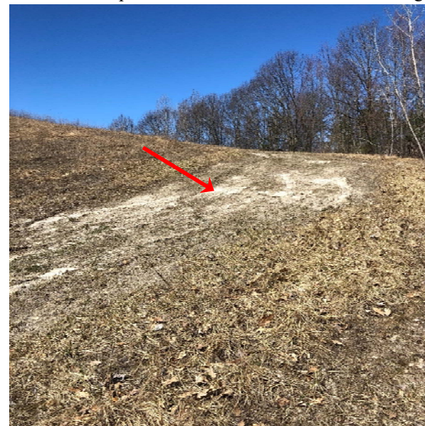
Photo #4: Erosion from vehicular traffic along southeast slope
