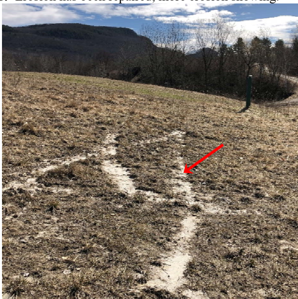
Photo #3: Erosion from vehicular traffic on south facing slope.
