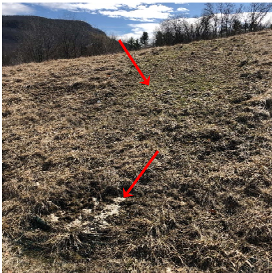
Photo #1: Erosion has been repaired, more erosion showing.
