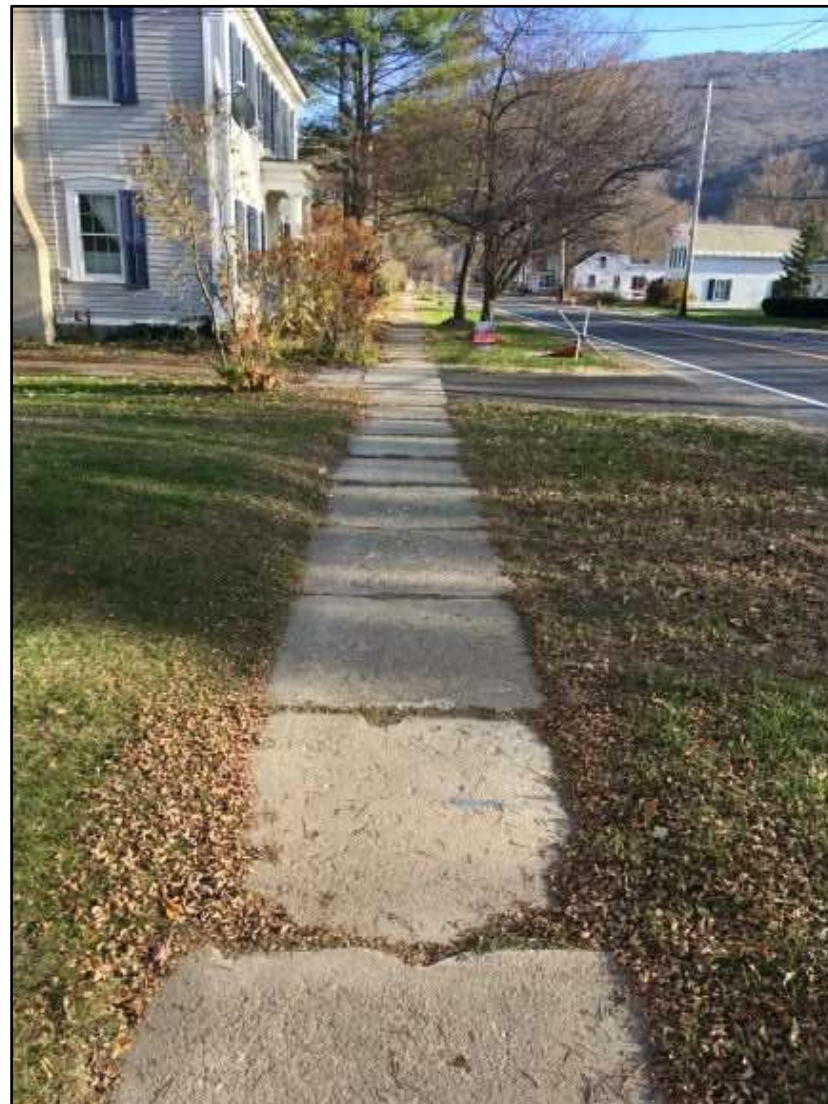
Figure 6. East Street looking eastward. (11/20/2020)
