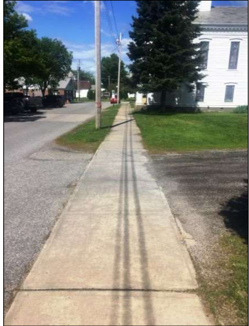
Figure 16. Park Place looking westward. (06/04/2019)
