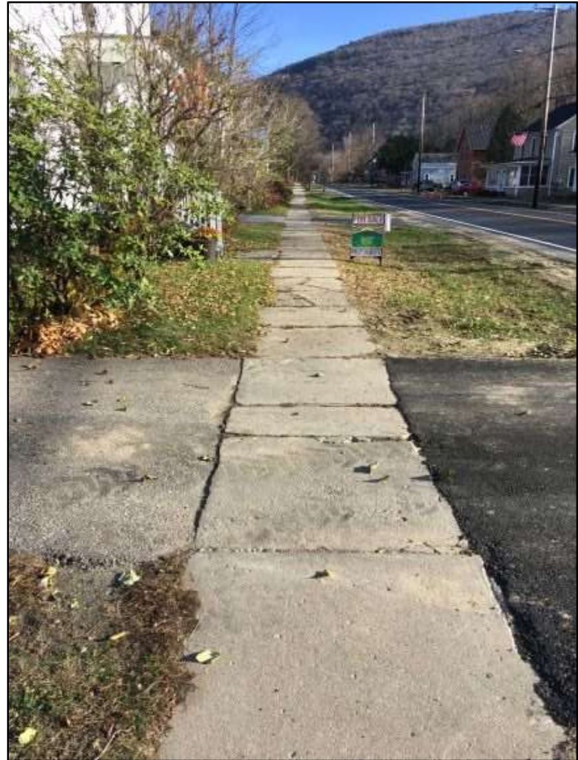
Figure 10. East Street looking eastward. (11/20/2020)
