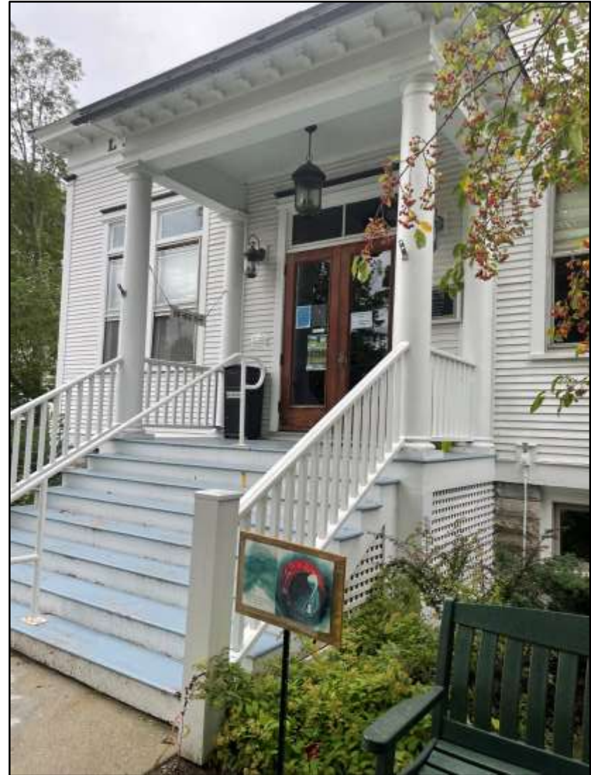
Figure 4. Front steps and porch, south side. (09/10/2021)
