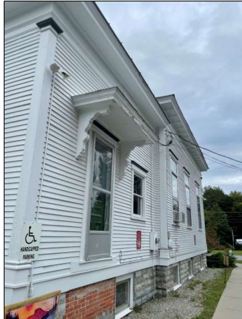
Figure 6. North side of the building. (09/10/2021)
