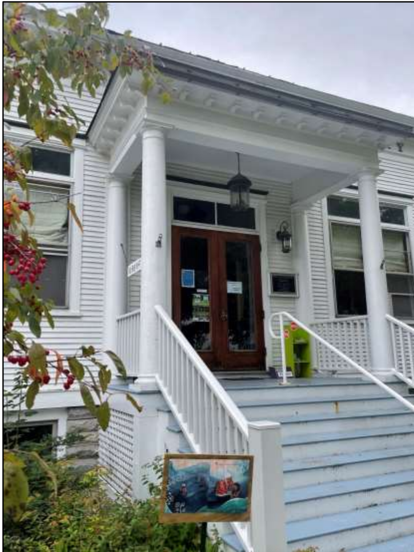
Figure 5. Front steps and porch, north side. (09/10/2021)
