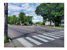
The existing pedestrian signals were upgraded with new ADA accessible push buttons and count-down pedestrian signal heads. Where needed, existing sidewalk ramps were replaced with ones having detectable warning surfaces. In addition, new crosswalks were added on the Plattsburg Avenue intersection (shown in the above photo) and the corner radii modified to reduce the length of the crosswalk across Plattsburg Avenue.
