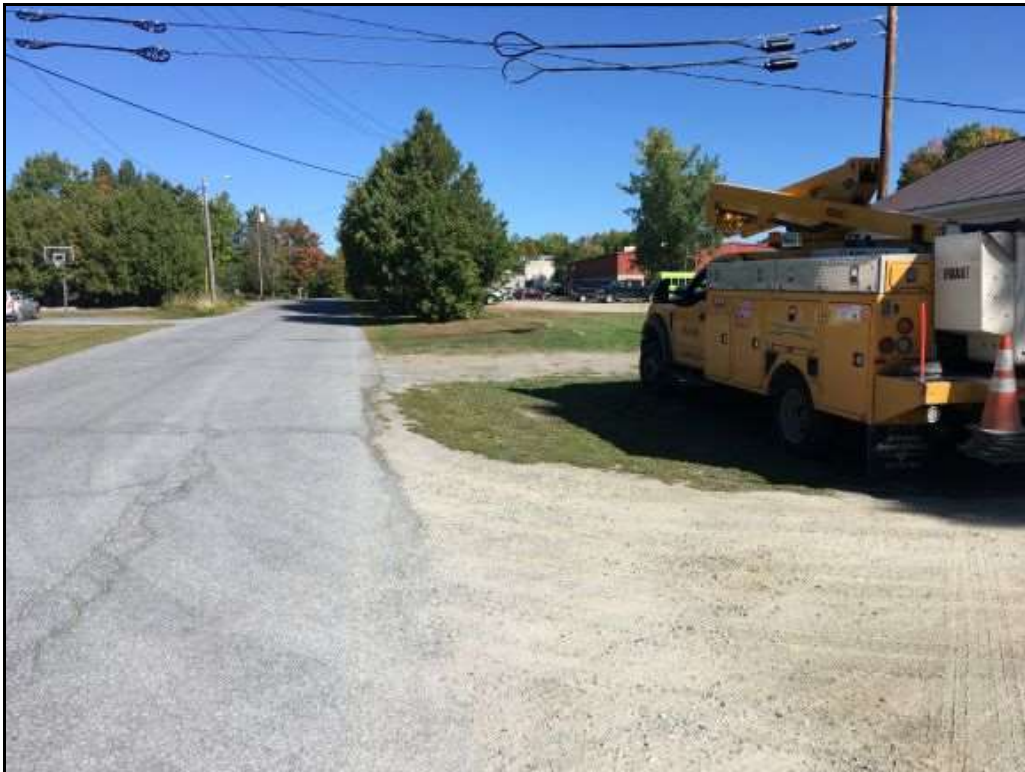
Figure 4. Munsill Avenue at WCVT substation south of Bristol Works. (09/18/2020)
