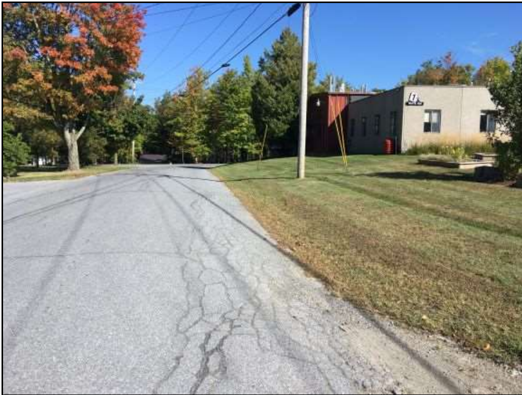
Figure 2. Munsill Avenue at Bristol Works near Pine Street intersection. (09/18/2020)
