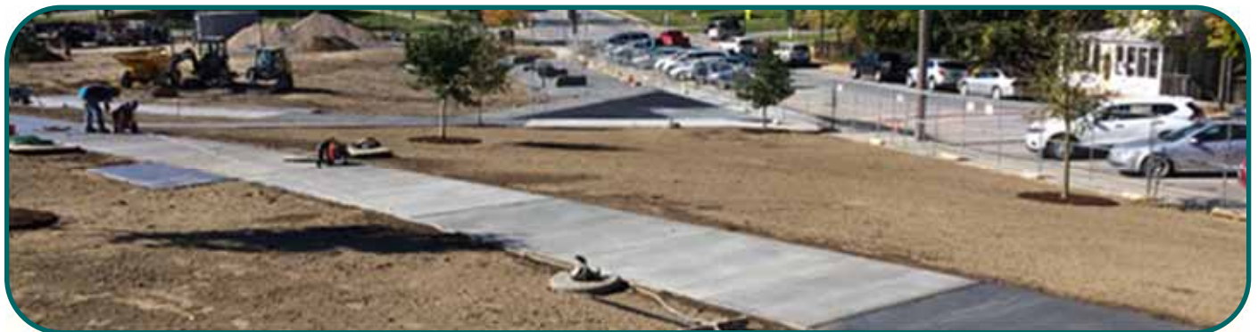
Sidewalk construction and the beginning of site restoration
