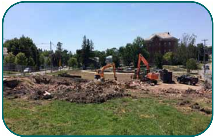
Excavation in the park
