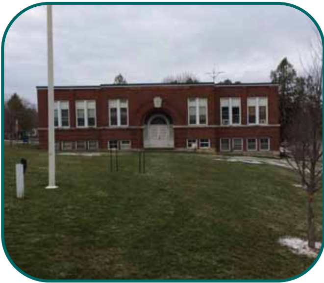
The now-demolished municipal offices
