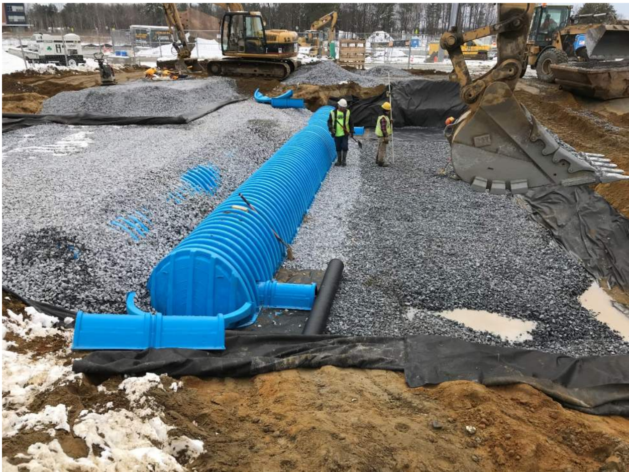
subsurface infiltration chamber system designed by EV during installation (March 2020)
