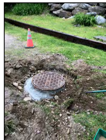
Repairs to dosing siphone manhole on South Street
