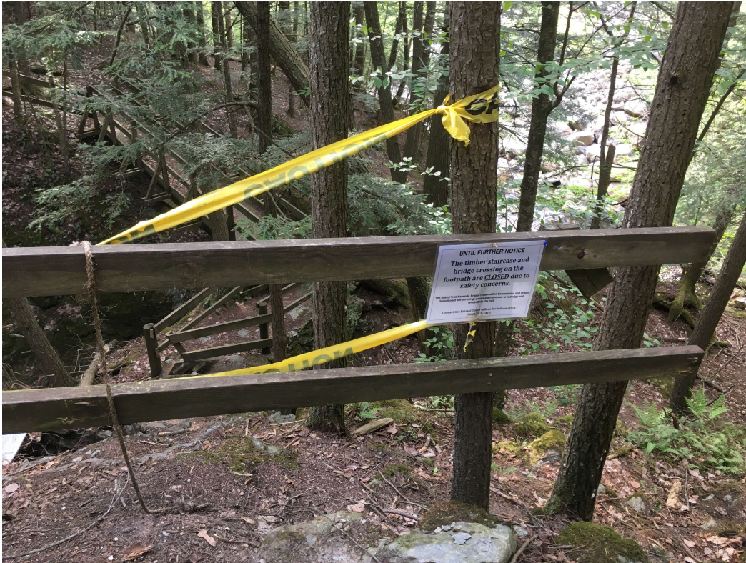
Figure 7. Signage, caution tape, and wooden planking mark the end of the footpath and closure of the bridge crossing at Memorial Park.
