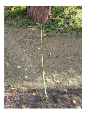
D. **Exhibit D**: Culvert placed at improper depth without cohesive soil plug. Proper depth is under 12 inches of soil with measures to stop further erosion into the culvert. Without further erosion mitigation measures this excessive taking of land will be pointless.
