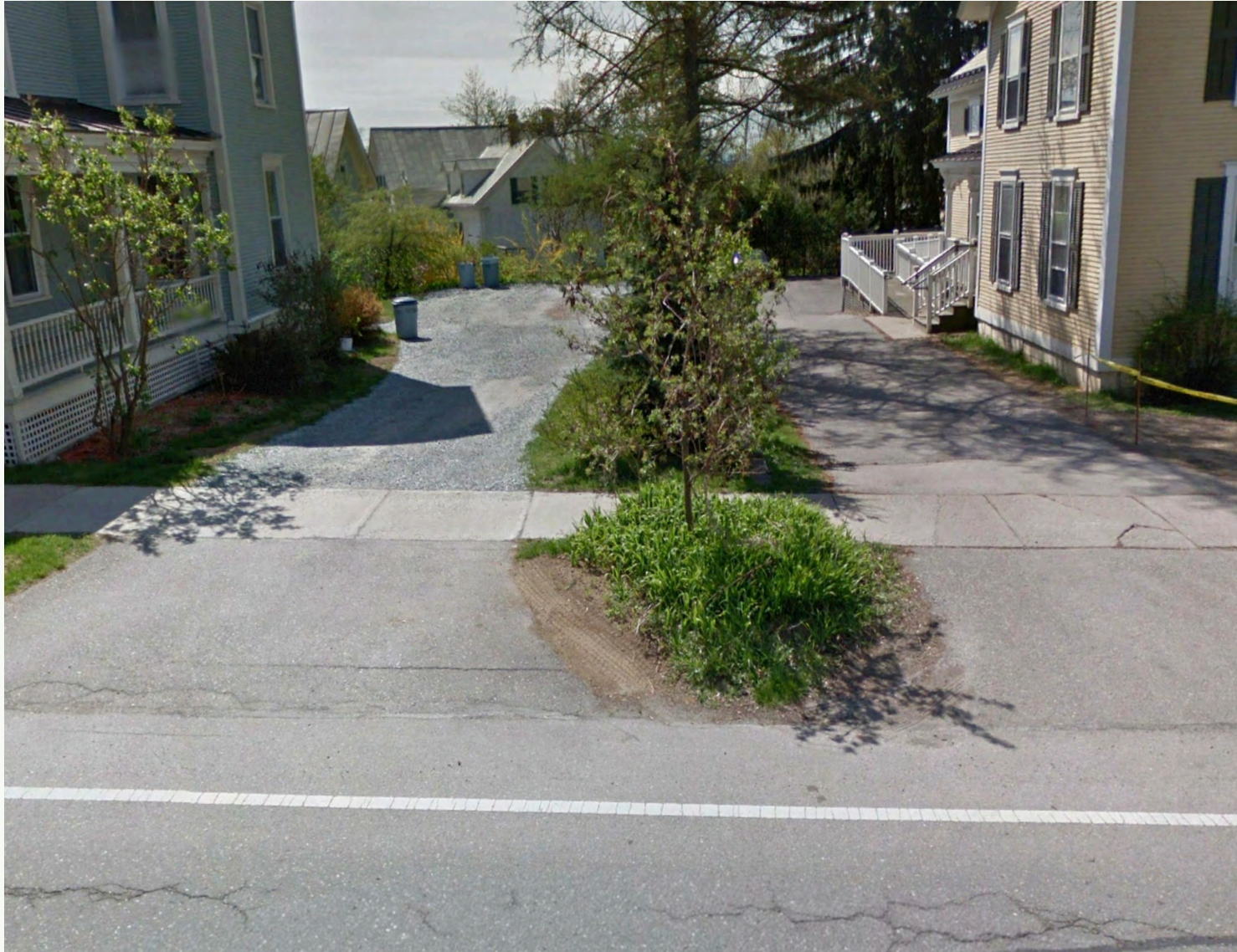
Continuous Flat Across Driveway
