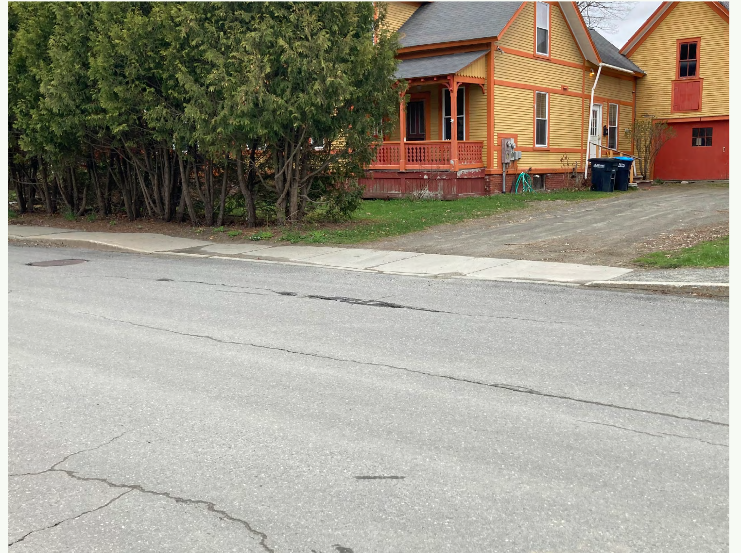
Continuous Dipped At Driveway - Curbed Condition Only
