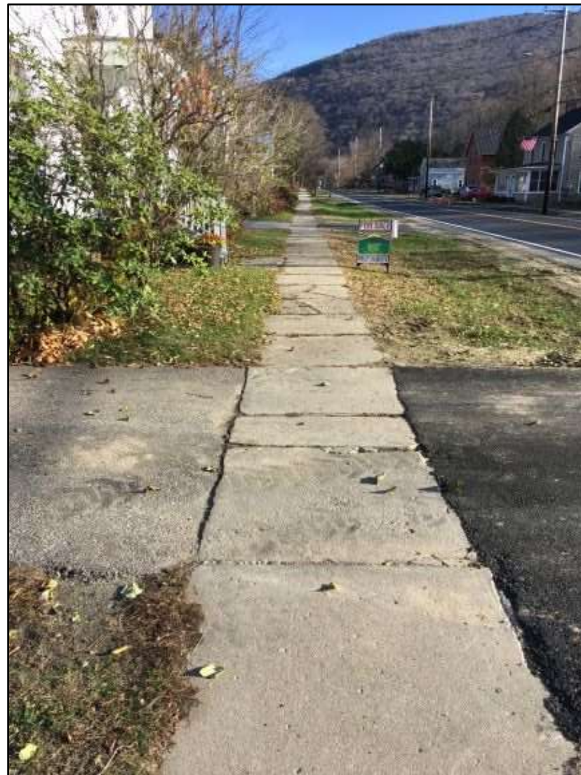
Figure 10. East Street looking eastward. (11/20/2020)
