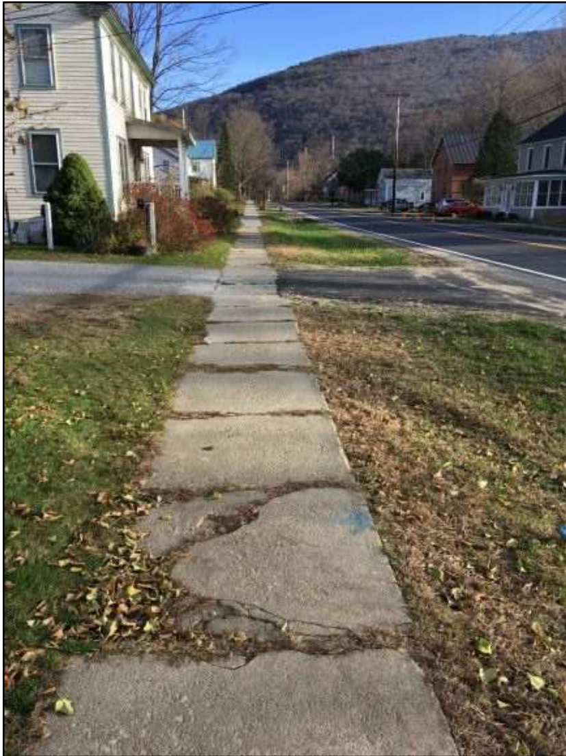
Figure 11. East Street looking eastward. (11/20/2020)
