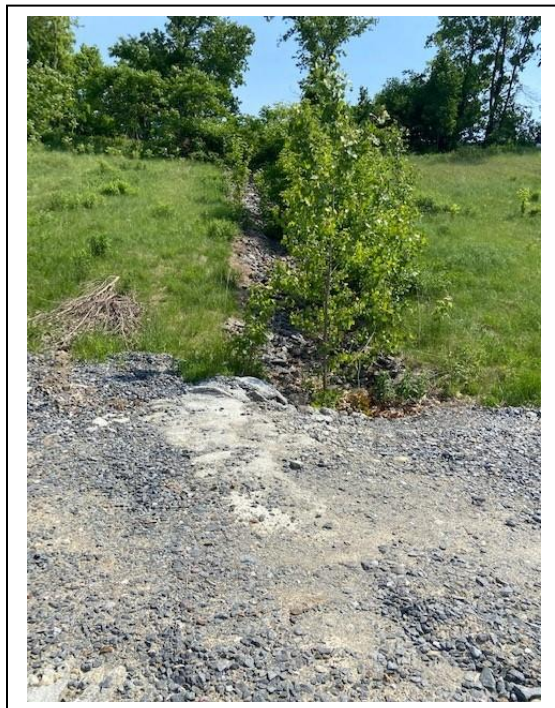
Photo #9 – Filled Stone Drainage Ditch & Growth
