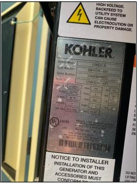
Brook Field Service and other bidders responded to the RFP that was based on the "bill of materials" from the original Generac generator calling for a PF of 0.8; however, the actual generator was built to 0.5 PF, as noted on the tag on the generator (above, left). The RFP also called for
