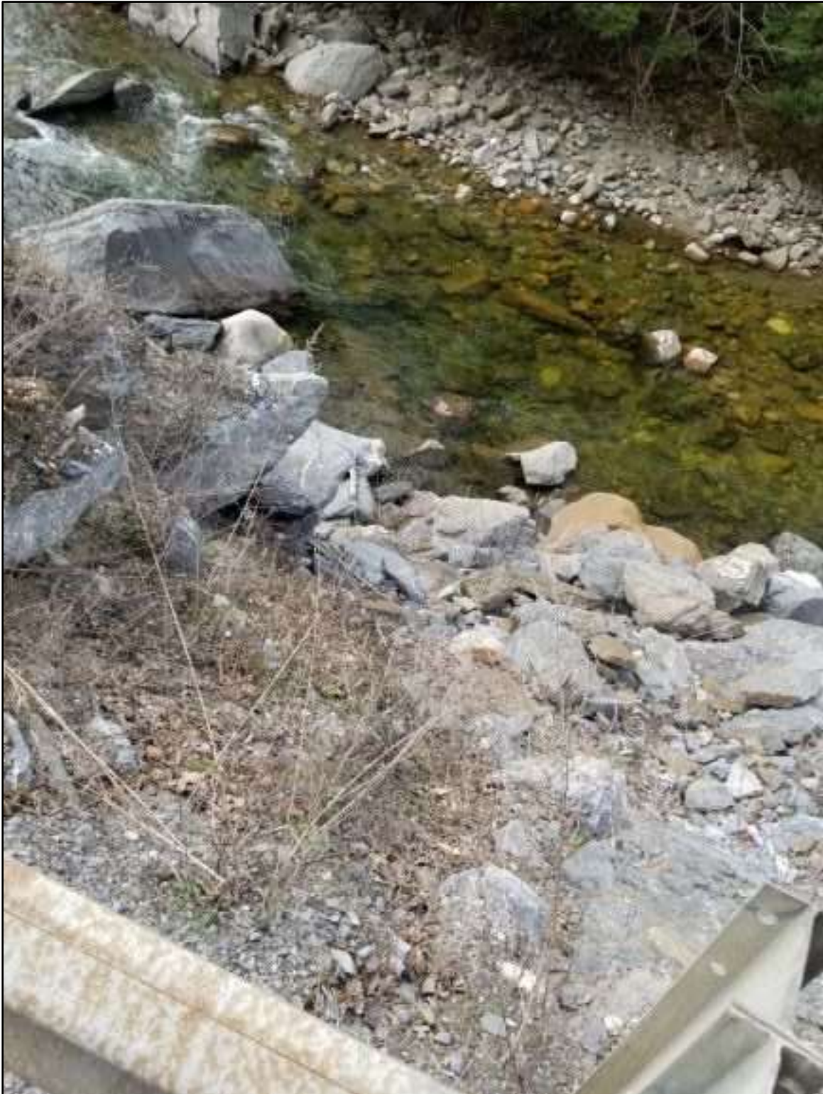
Figure 3. View of the newer slide from the shoulder. (Photo: Cota)
