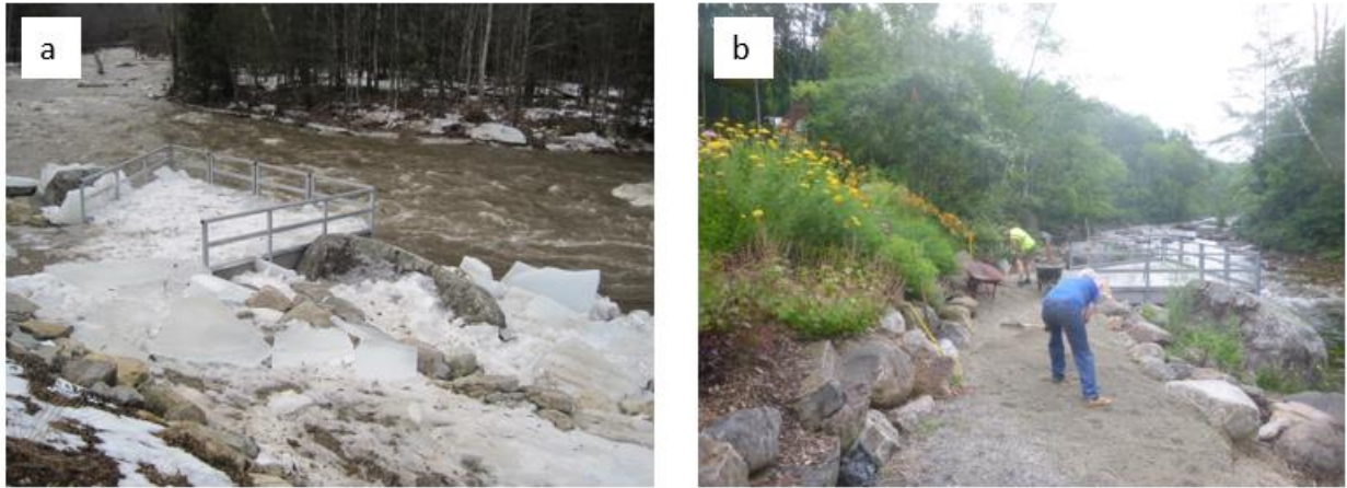
Figure 6. Universal Fishing Platform (a) receives ice during thaw event on January 30, 2013. (b) Bristol CC members replace gravel on access ramp to the platform during an August repair activity following flooding on July 1, 2017 that eroded a segment of the walkway.
