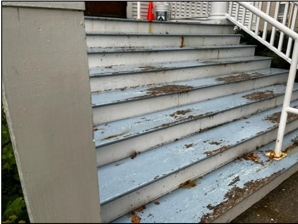
Figure 3. Closer view of the Lawrence Memorial Library front steps (Mosely, 08/15/2022).
