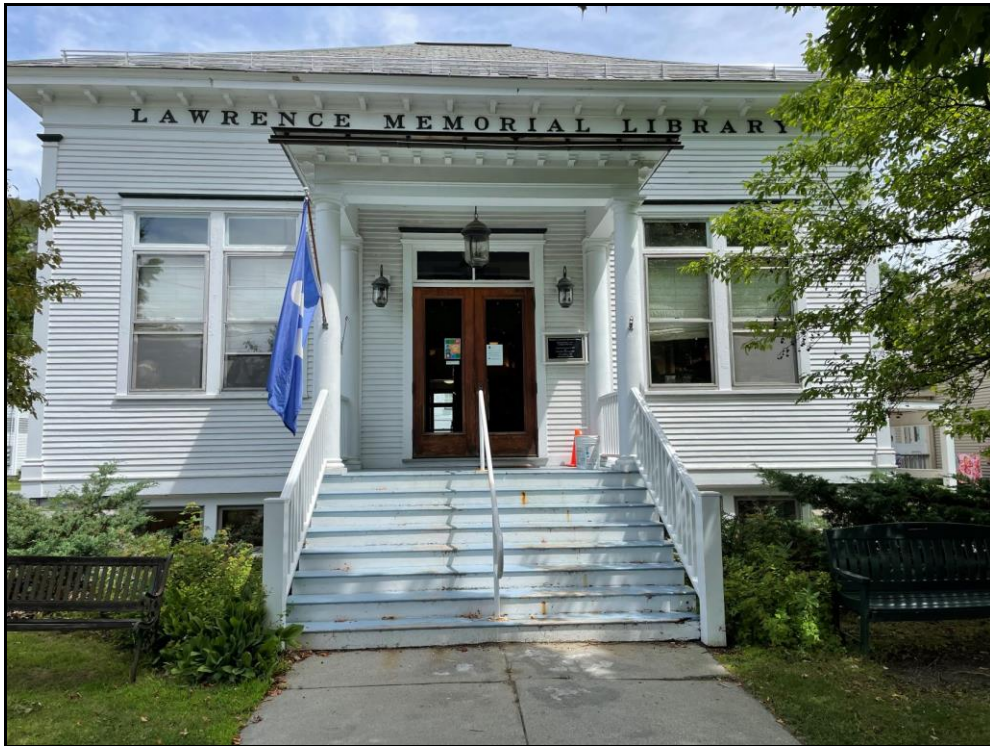
Figure 1. Lawrence Memorial Library front entry west side (07/27/2022).
