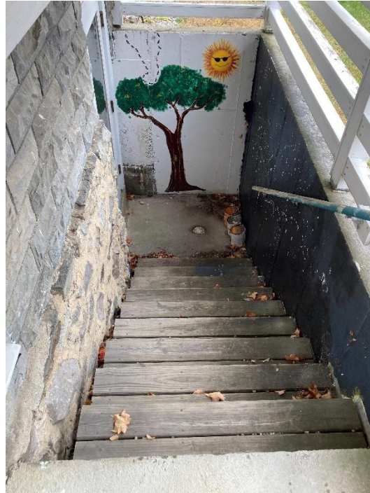
Figure 16a- Egress door and stairs from lower level (outside)
