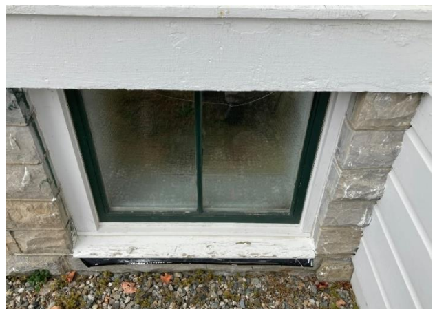
Figure 18b- Lower-level bathroom window
