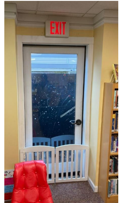
Figure 16b- Egress door and stairs from lower level (inside)
