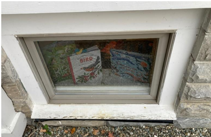
Figure 18a- Typical lower-level Al. clad wood window
