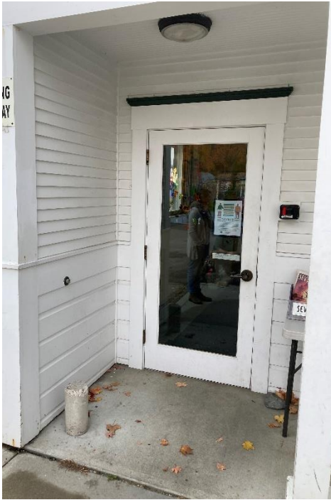
Figure 15- ADA entrance on the North side
