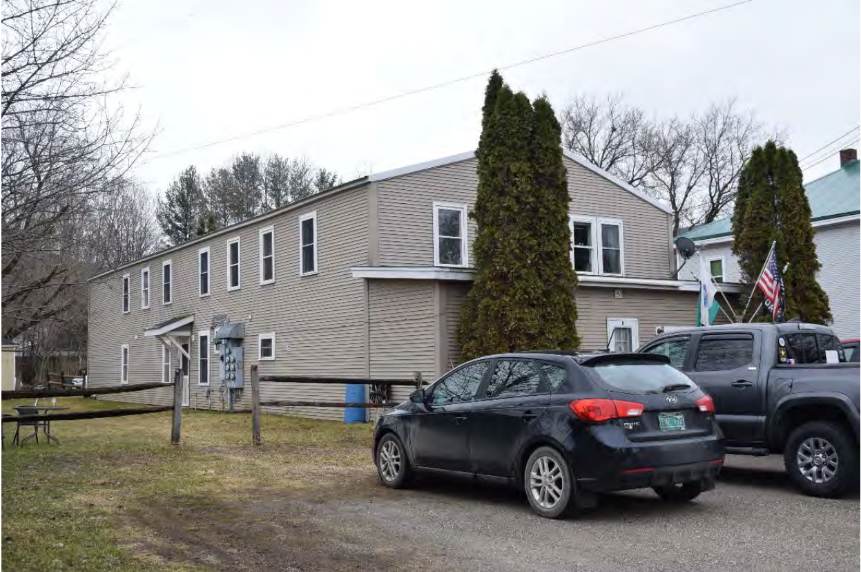
Photo 54. View of Structure 20 at 42 Munsill Avenue, looking east-southeast.
