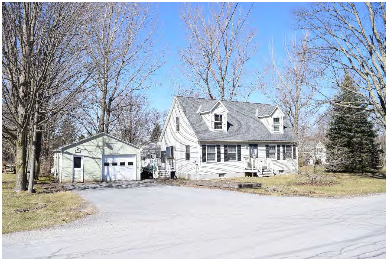
Photo 7. View of Structure 2 at 79 Munsill Avenue, looking northwest.
