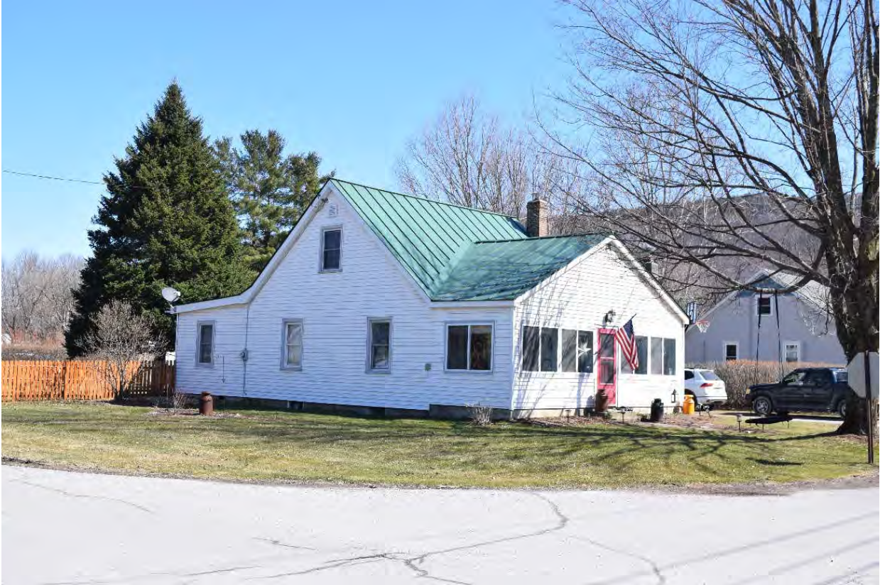
Photo 58. View of Structure 22 at 58 West Pleasant Street, looking northeast.
