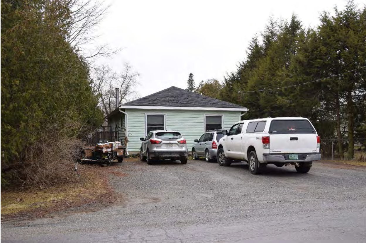
Photo 19. View of Structure 6 at 63 Munsill Avenue, facing west-northwest.
