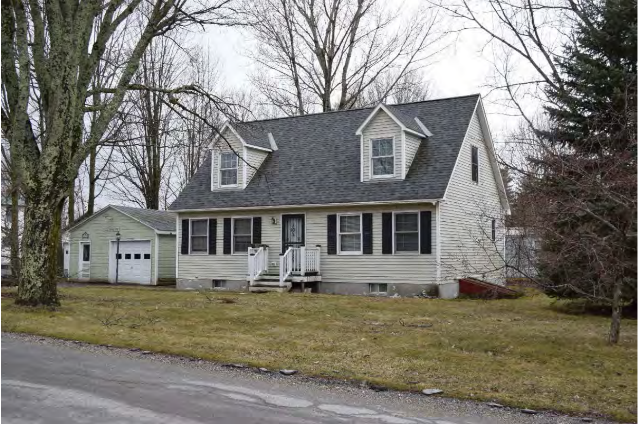
Photo 8. View of Structure 2 at 79 Munsill Avenue, facing southwest.
