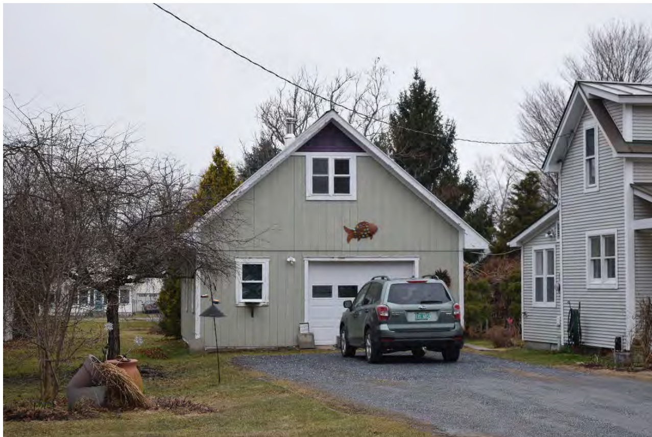
Photo 17. View of garage associated with Structure 5, looking west.
