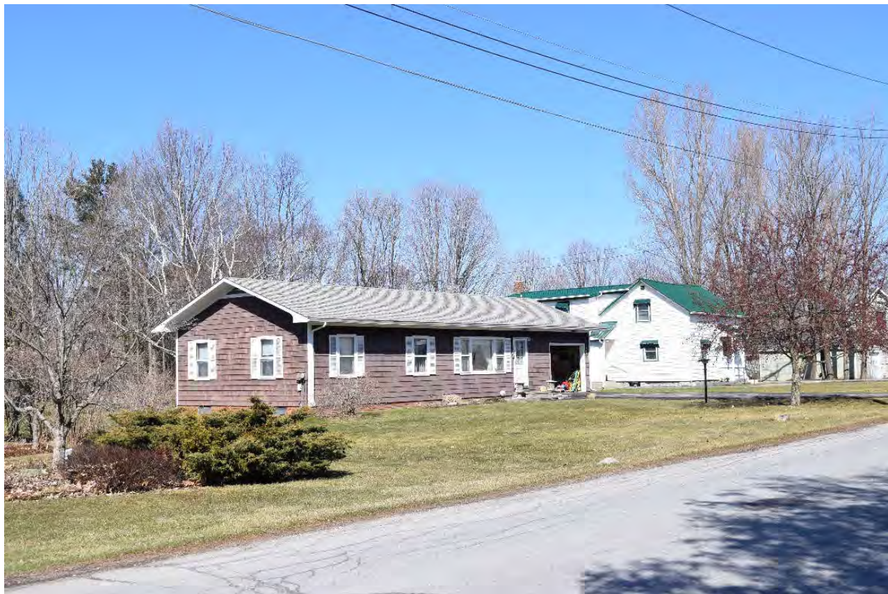
Photo 14. View of Structure 4 at 71 Munsill Avenue, facing northwest.
