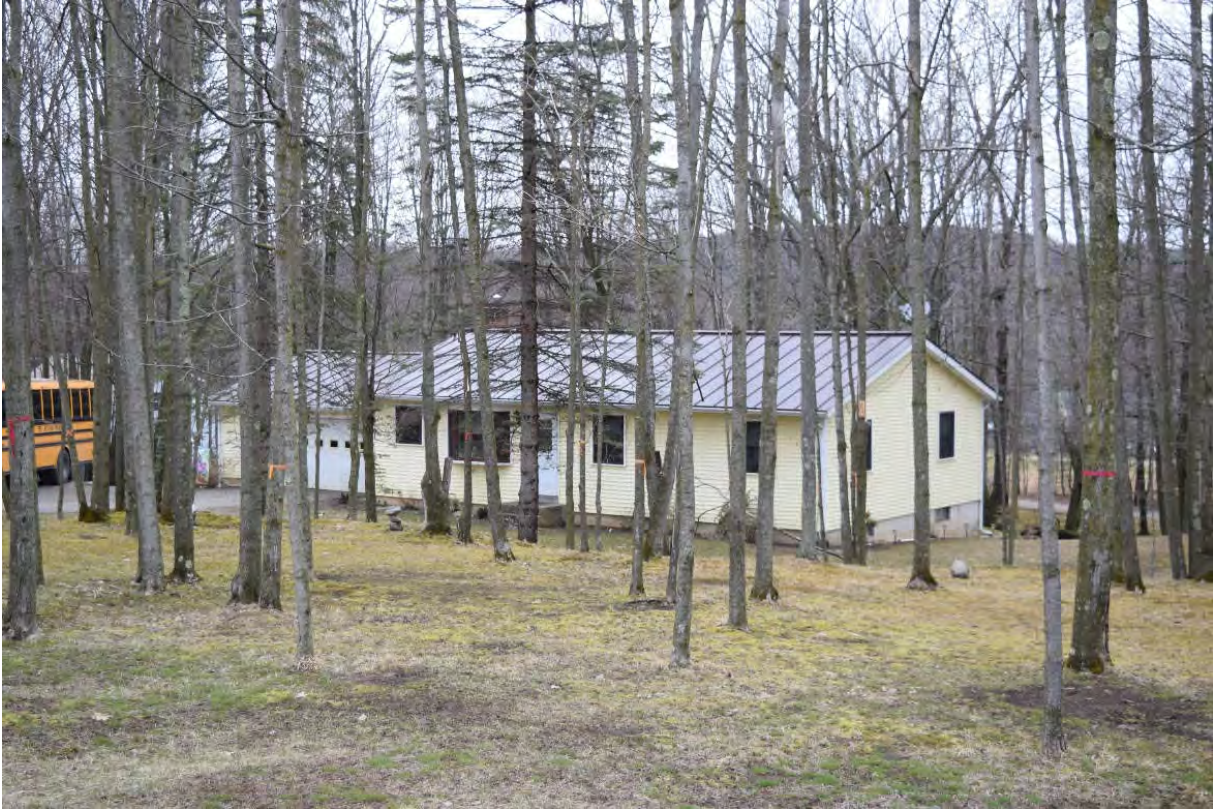
Photo 6. View of Structure 1 at 60 Pine Street, looking north-northwest.
