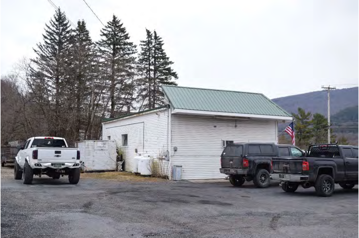
Photo 44. View of Structure 16 at 58 West Street, facing southeast.
