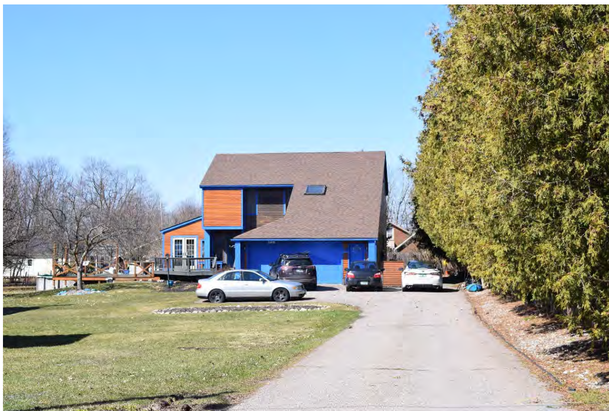
Photo 20. View of Structure 7, facing west-southwest.
