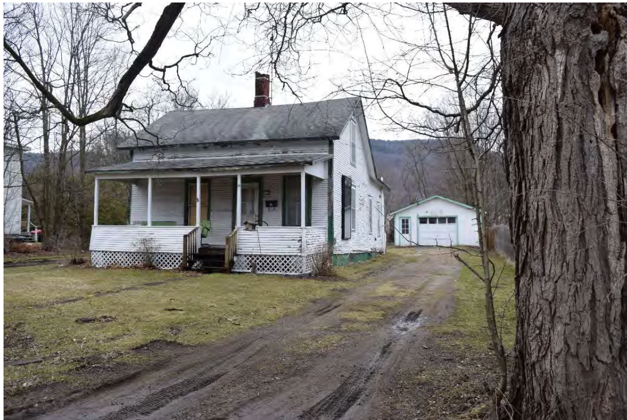
Photo 45. View of Structure 17 at 20 Munsill Avenue, looking east-northeast.
