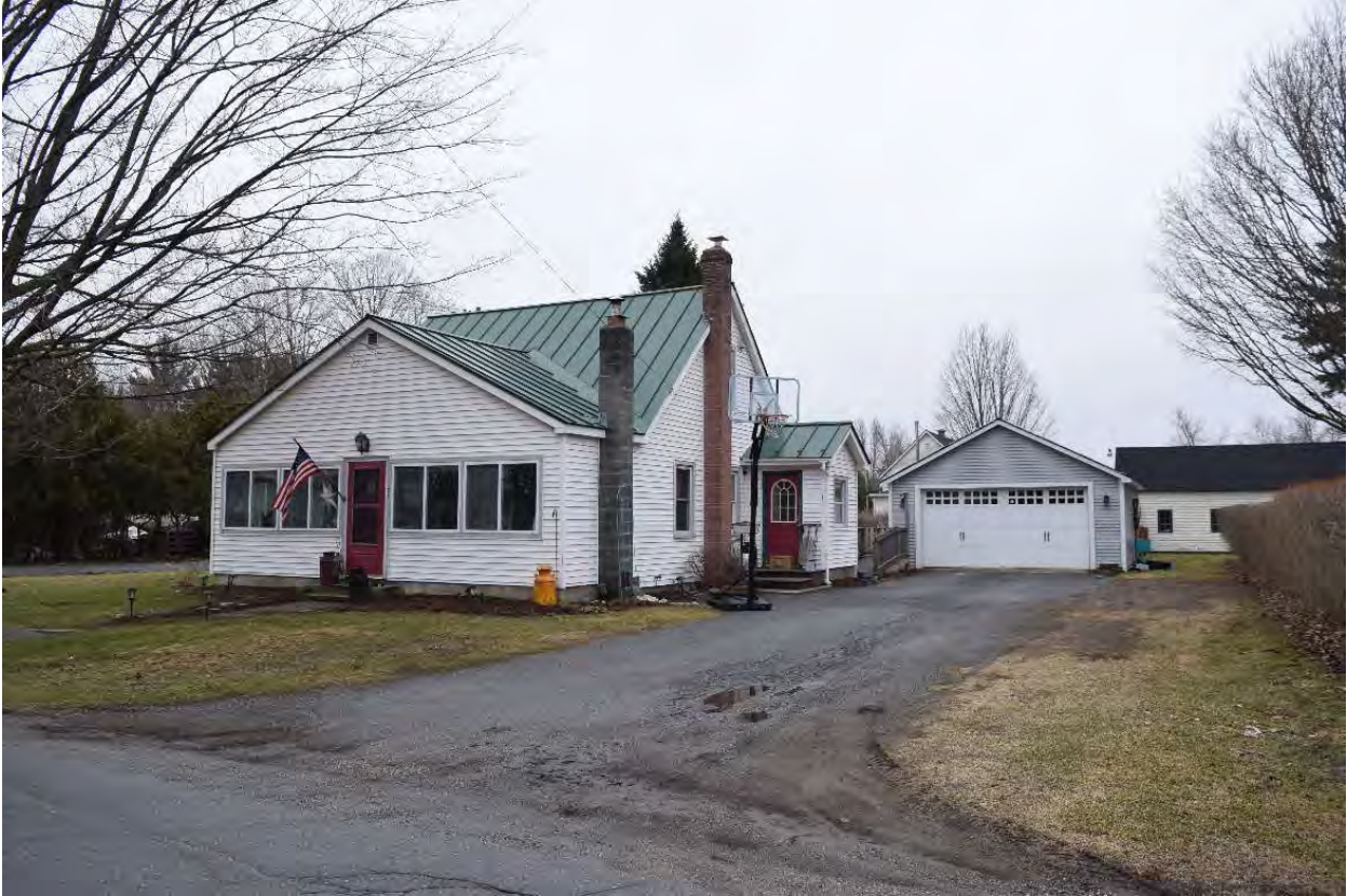
Photo 57. View of Structure 22 at 58 West Pleasant Street, looking north-northwest.
