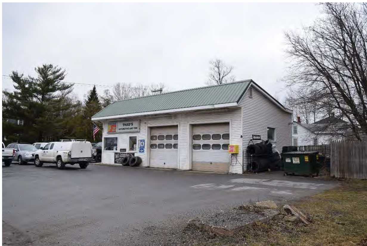
Photo 42. View of Structure 16 at 58 West Street, looking northwest.
