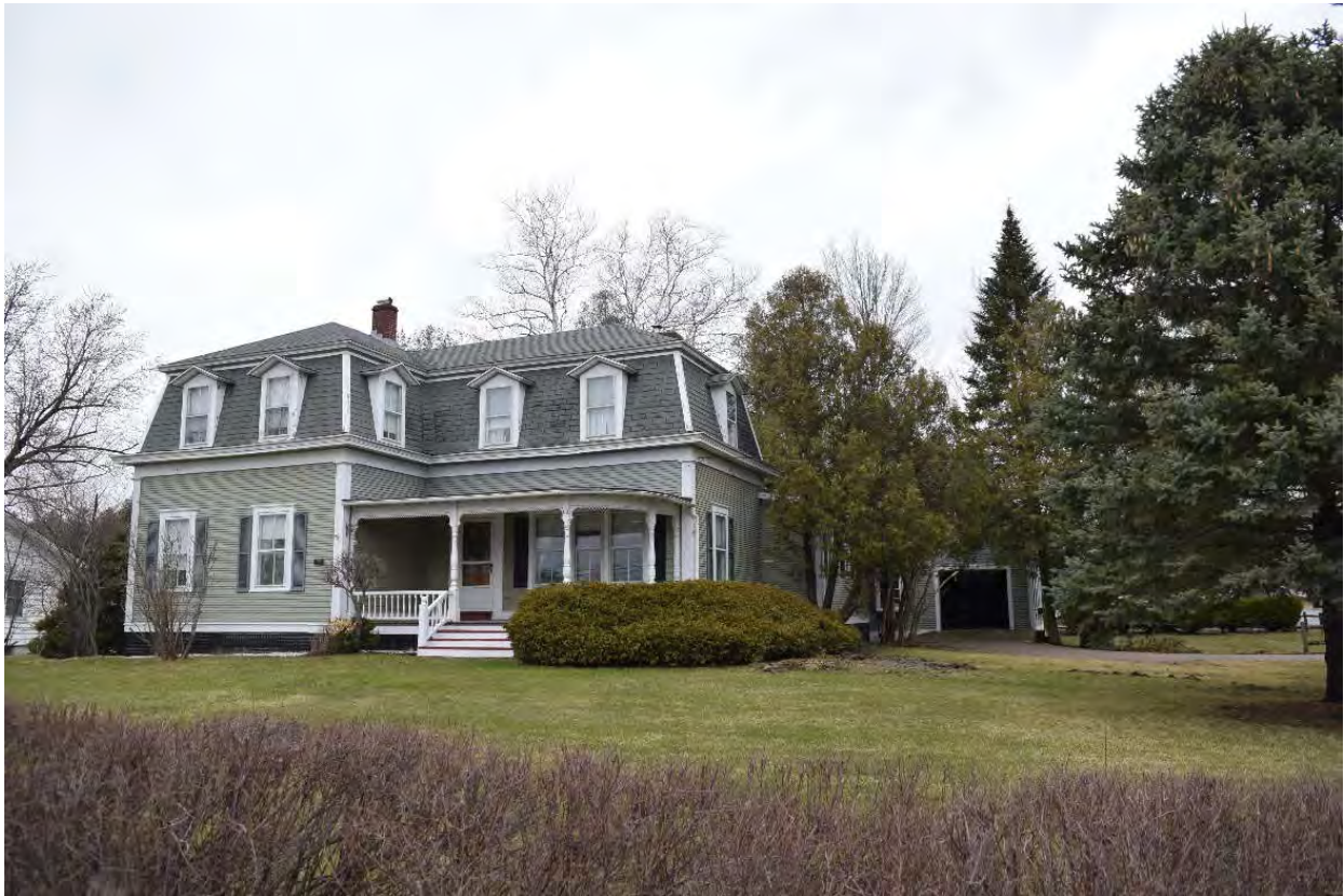
Photo 39. View of Structure 15 at 60 West Street, looking northwest.
