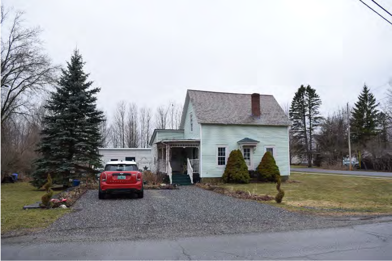
Photo 29. View of Structure 11 at 49 Munsill Avenue, facing west.
