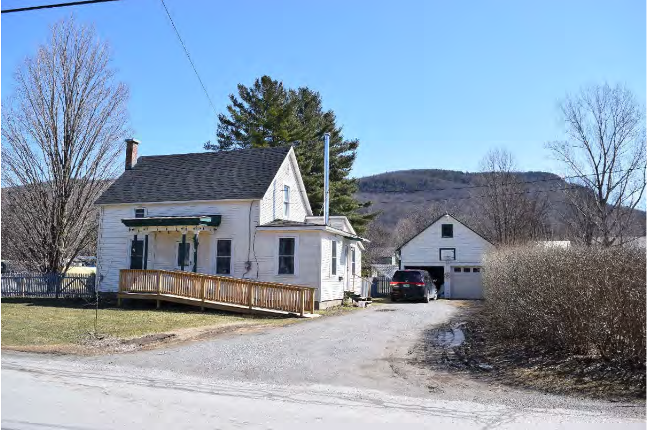
Photo 60. View of Structure 23 at 54 Munsill Avenue, looking east-northeast.
