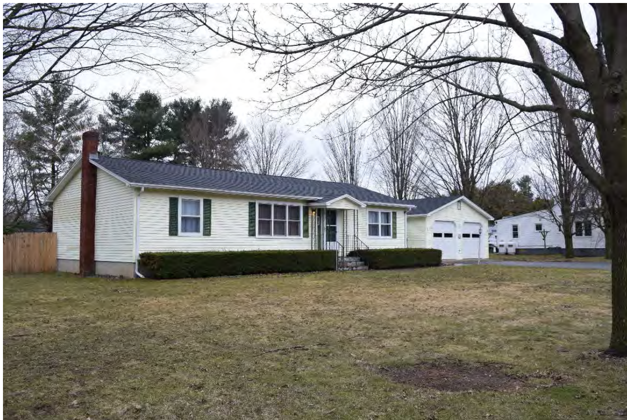
Photo 25. View of Structure 9 at 57 Munsill Avenue, looking northwest.
