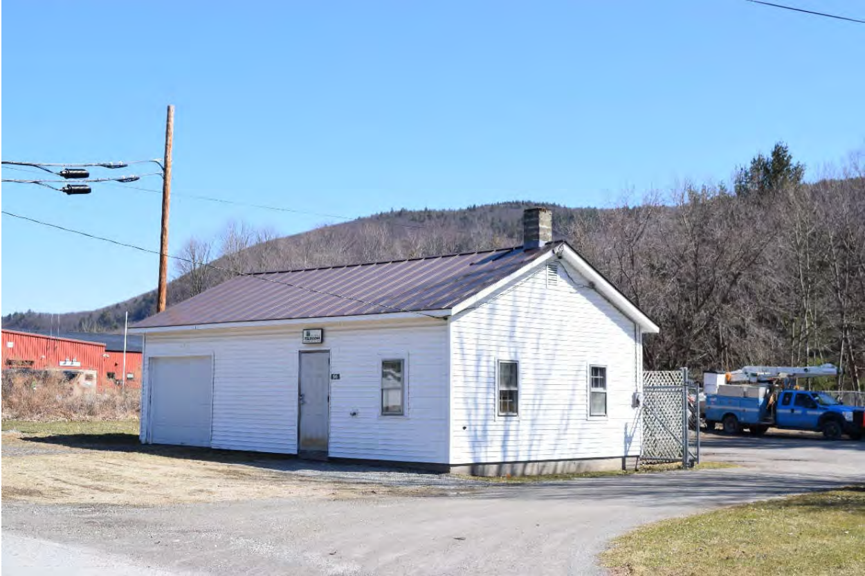
Photo 63. View of Structure 24 at 56 Munsill Avenue, looking northeast.
