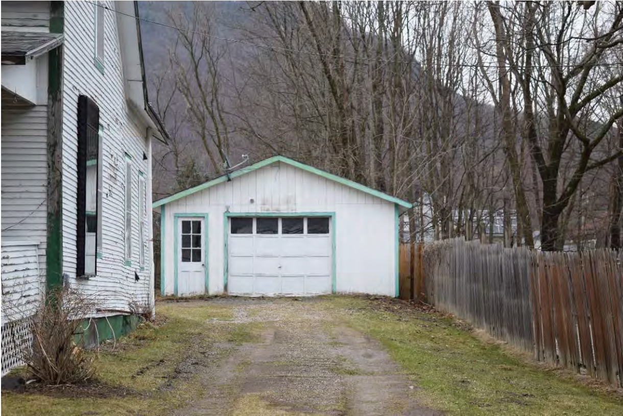
Photo 47. View garage associated with Structure 17 at 20 Munsill Avenue, looking east.
