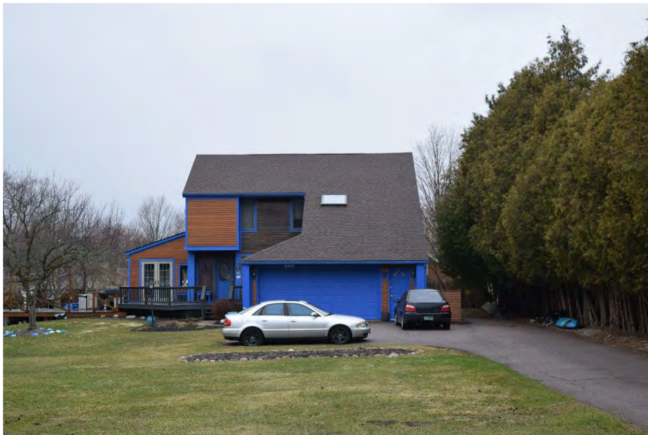
Photo 21. View of Structure 7, facing west.
