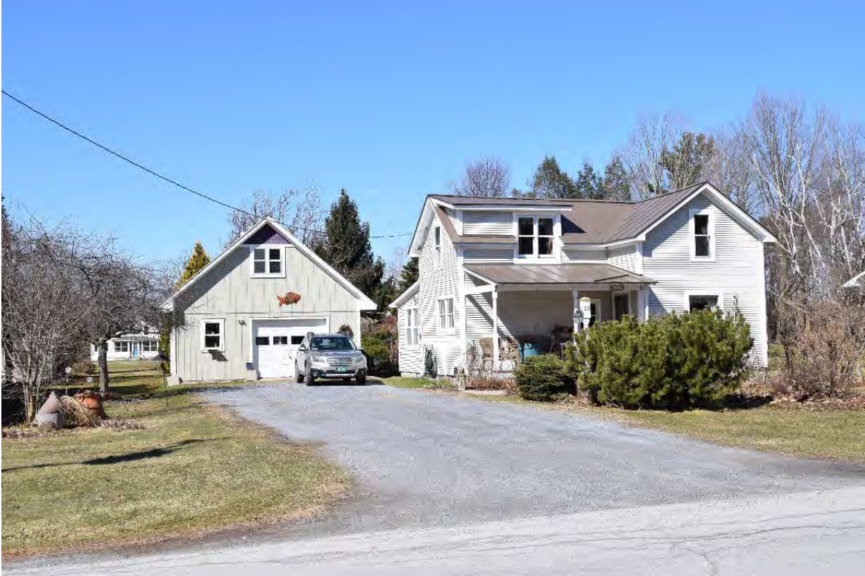
Photo 15. View of Structure 5 at 65 Munsill Avenue, facing west-northwest.
