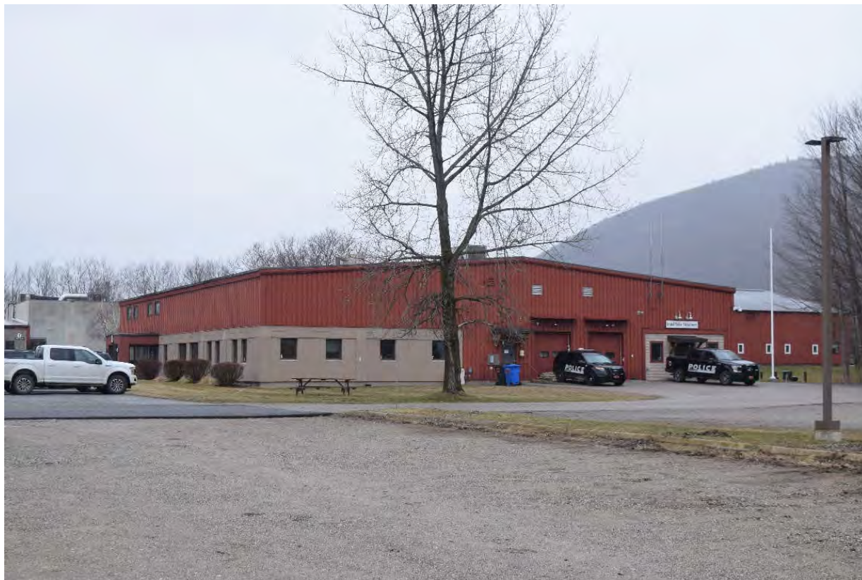
Photo 67. View of south building in the Structure 25 complex (72 Munsill Avenue), looking northeast.
