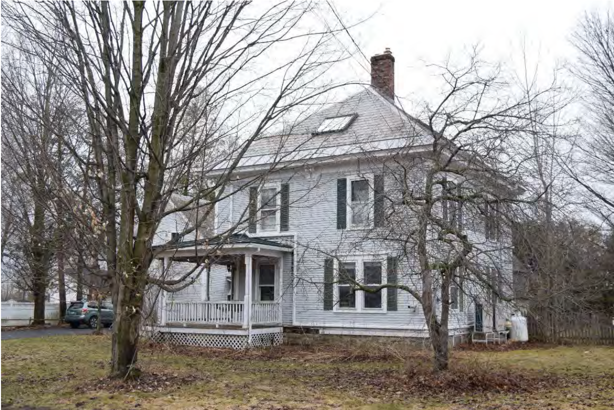
Photo 37. View of Structure 14 at 21 Munsill Avenue, looking west-southwest.
