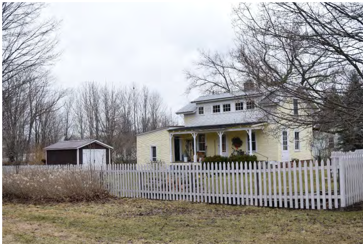
Photo 31. View of Structure 12 at 43 Munsill Avenue, facing northwest.
