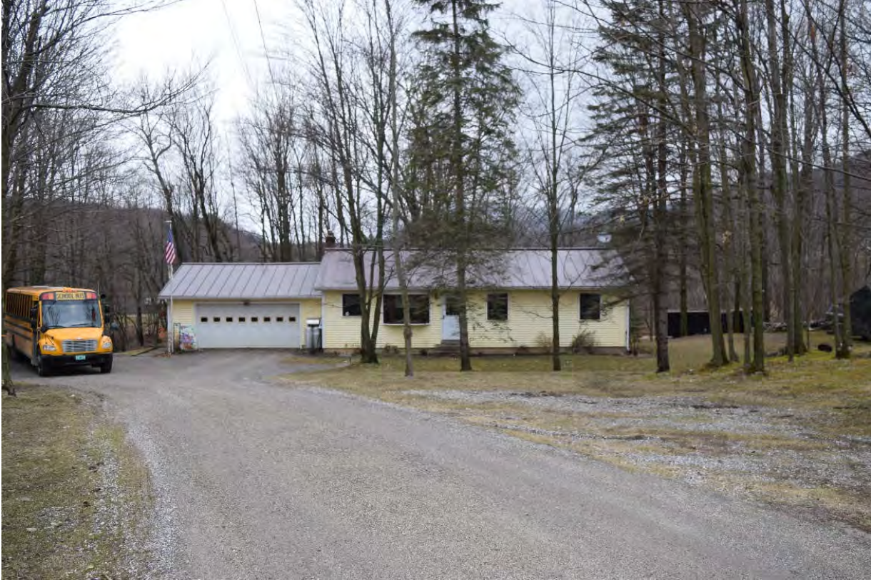
Photo 5. View of Structure 1 at 60 Pine Street, facing north.
