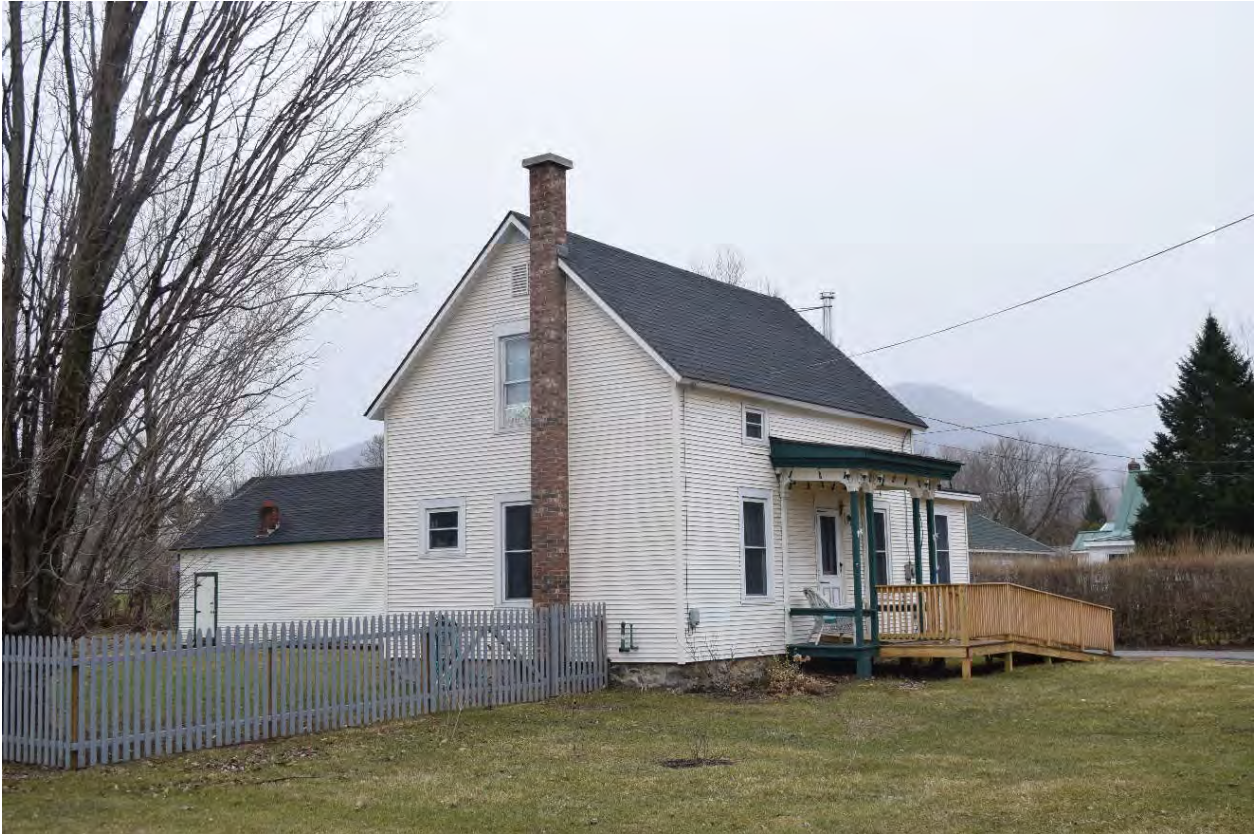
Photo 61. View of Structure 23 at 54 Munsill Avenue, looking southeast.
