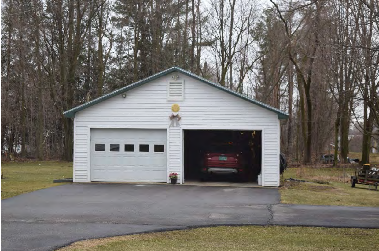
Photo 12. View of garage associated with Structure 3 at 73 Munsill Avenue, looking west.
