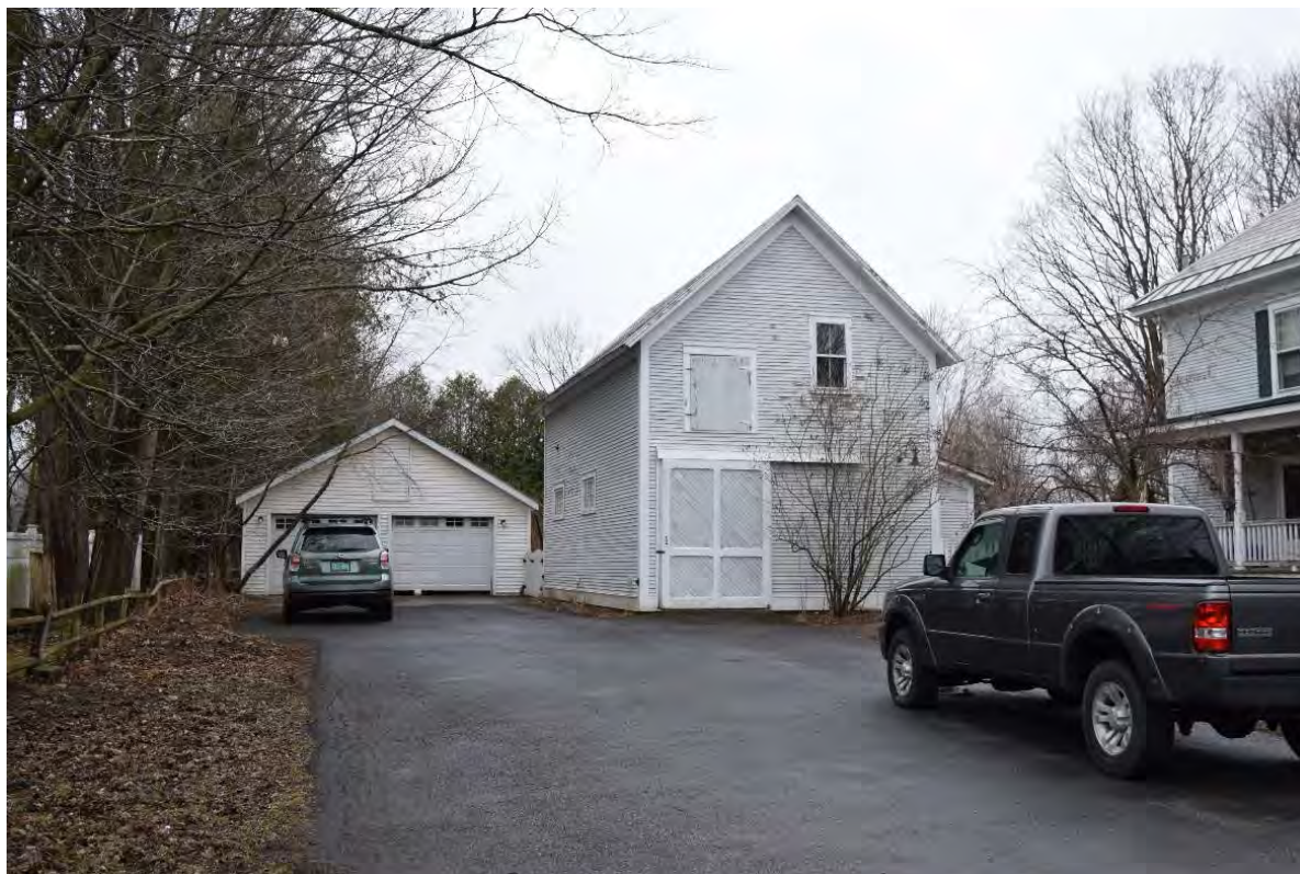
Photo 38. View of buildings associated with Structure 14 at 21 Munsill Avenue, looking west.
