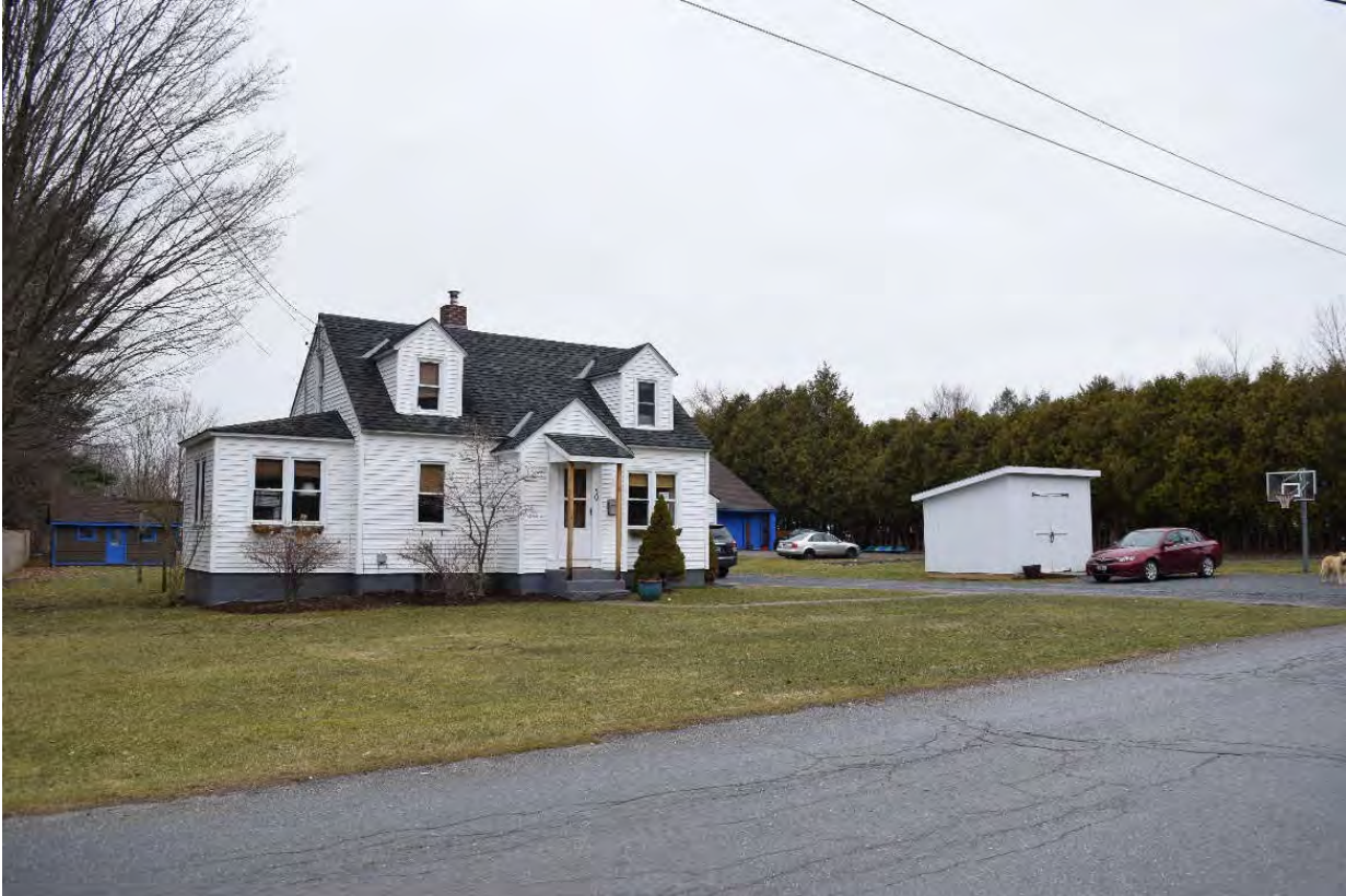
Photo 23. View of Structure 8 at 59 Munsill Avenue, looking northwest.
