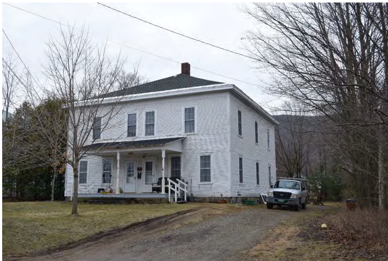
Photo 48. View of Structure 18 at 28-30 Munsill Avenue, looking northeast.
