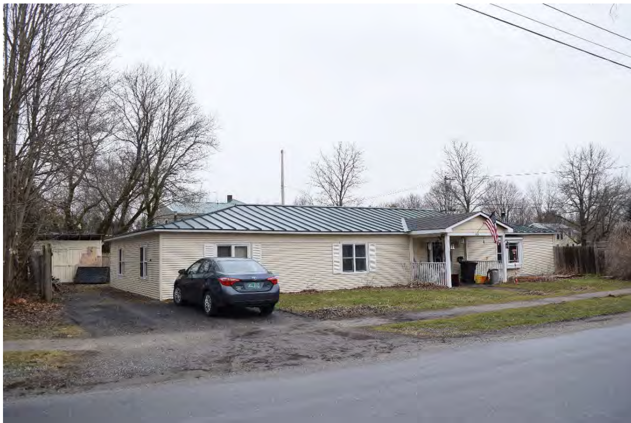
Photo 55. View of Structure 21 at 55 West Pleasant Street, looking southwest.
