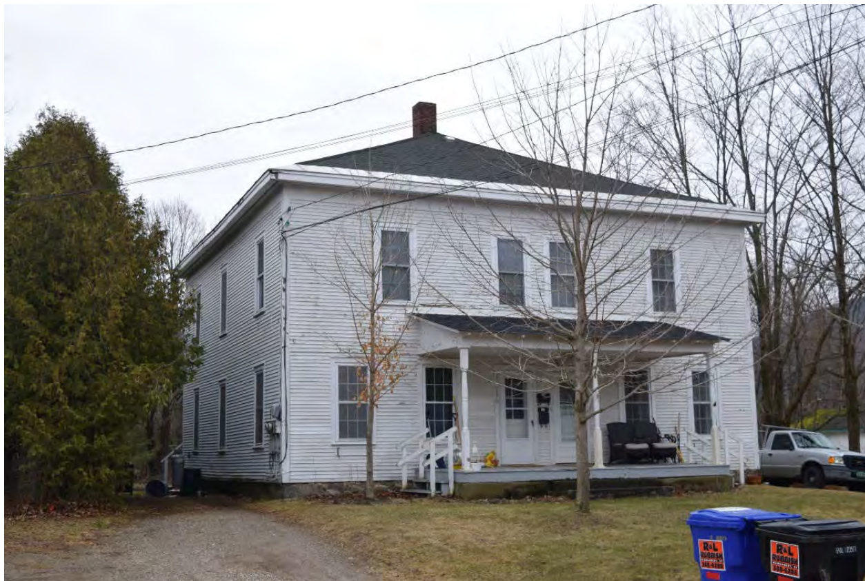
Photo 49. View of Structure 18 at 28-30 Munsill Avenue, facing east-southeast.
