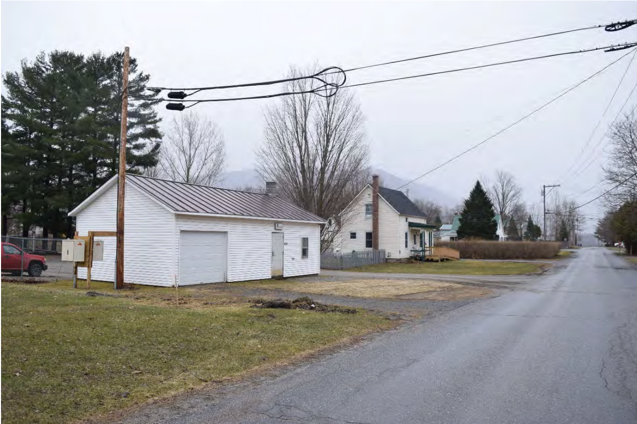
Photo 64. View of Structure 24 at 56 Munsill Avenue, looking south-southeast.
