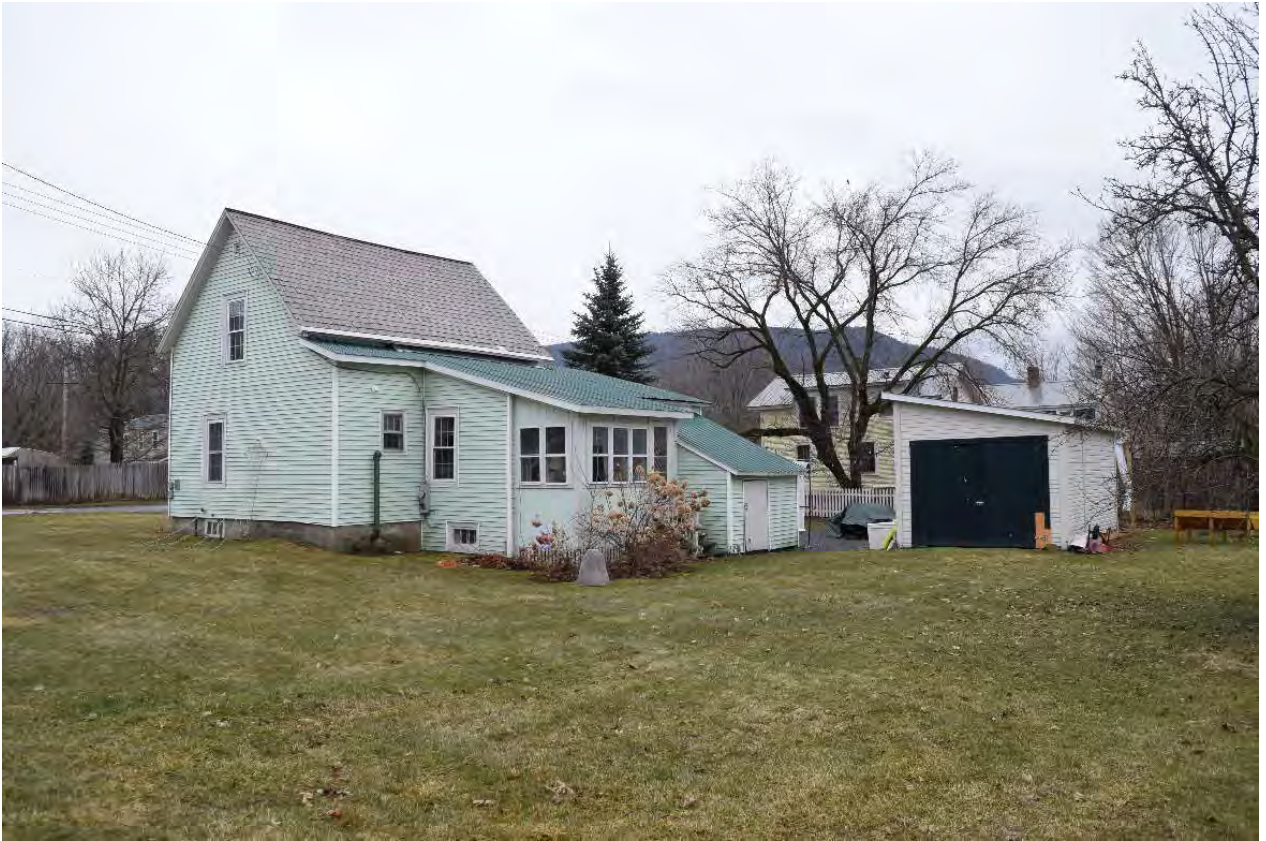
Photo 30. View of Structure 11 at 49 Munsill Avenue, facing southeast.
