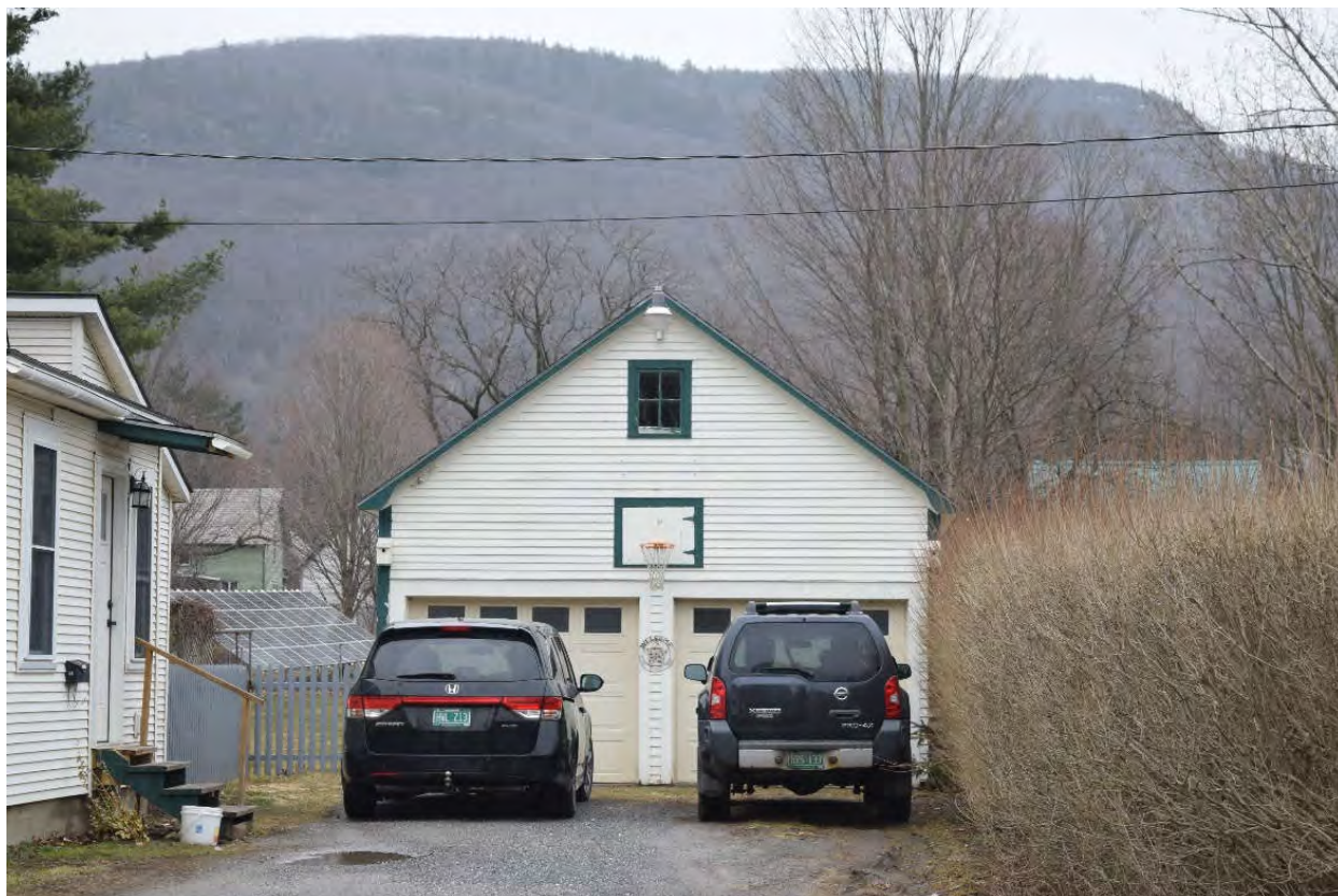
Photo 62. View of building associated with Structure 23, looking east.
