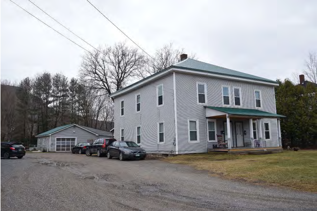
Photo 50. View of Structure 19 at 36 Munsill Avenue, looking southeast.
