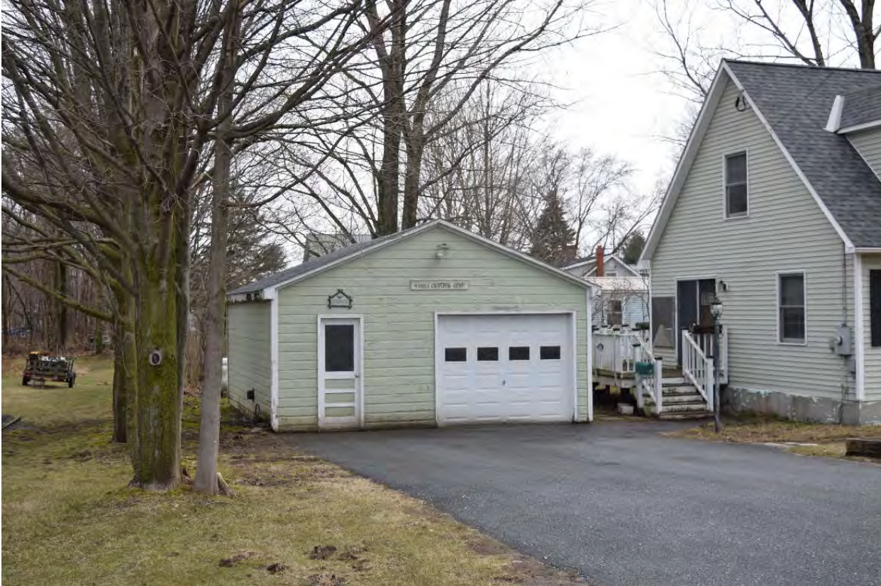
Photo 9. View of garage associated with Structure 2, facing west.
