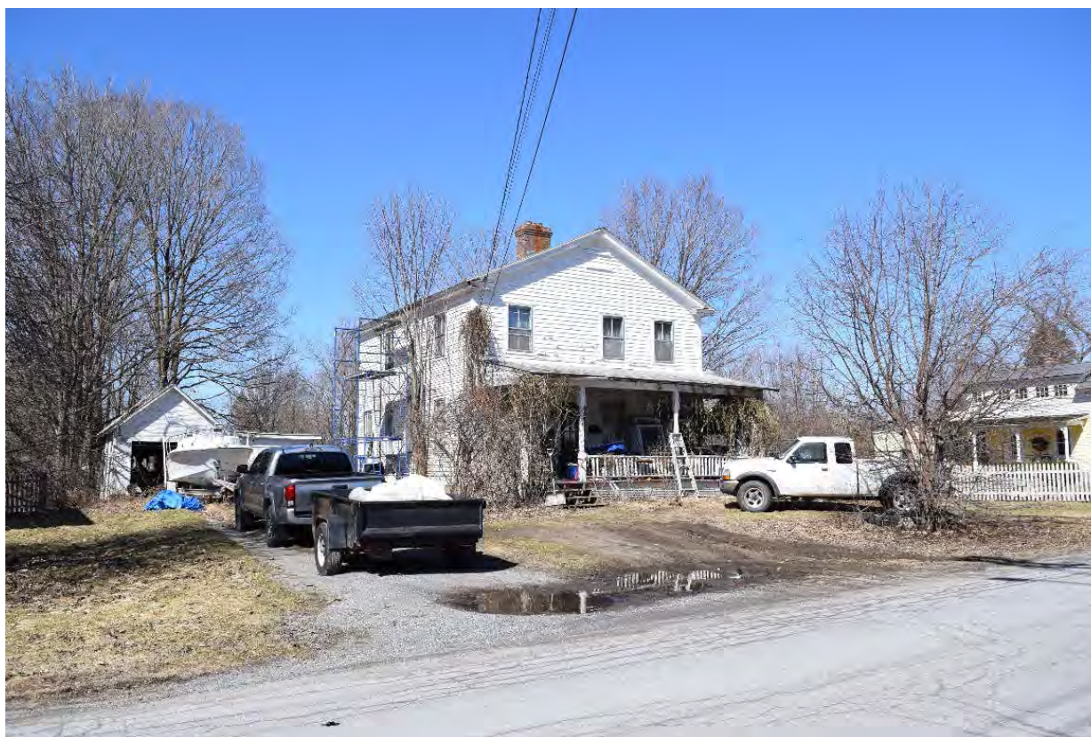
Photo 34. View of Structure 13 at 31 Munsill Avenue, looking northwest.
