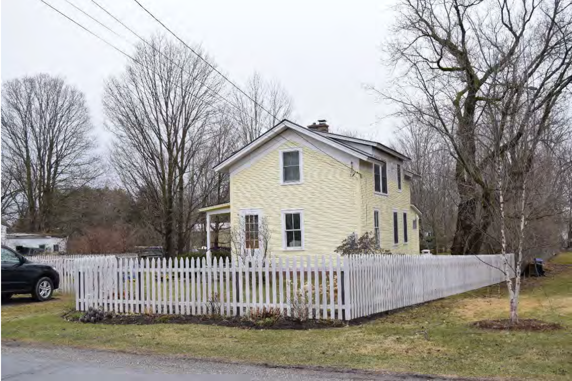
Photo 32. View of Structure 12 at 43 Munsill Avenue, facing west-southwest.
