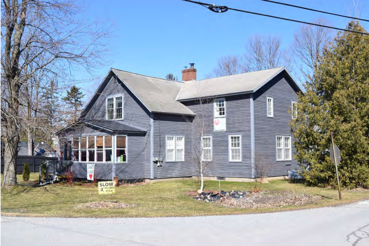
Photo 26. View of Structure 10 at 60 West Pleasant Street, facing northwest.
