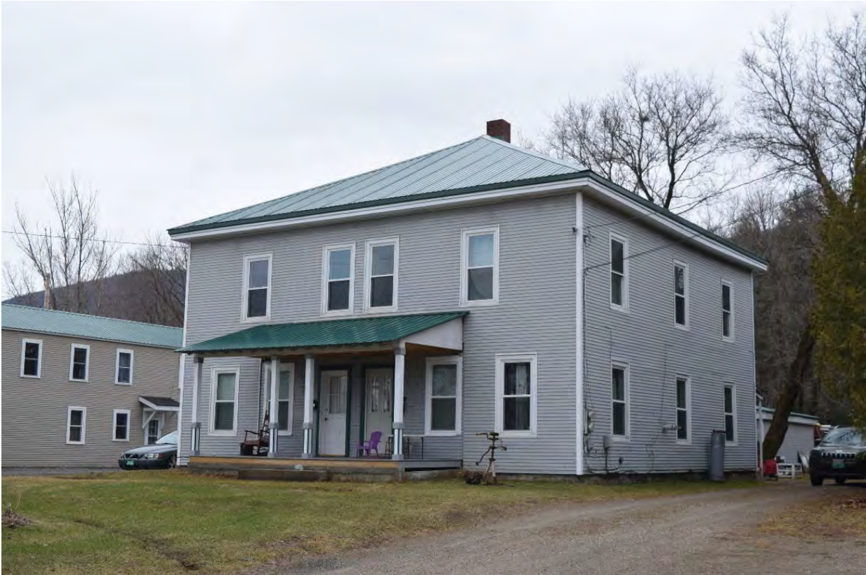
Photo 51. View of Structure 19 at 36 Munsill Avenue, facing northeast.
