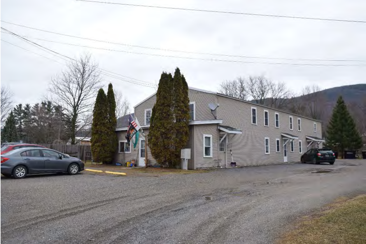
Photo 53. View of Structure 20 at 42 Munsill Avenue, looking northeast.
