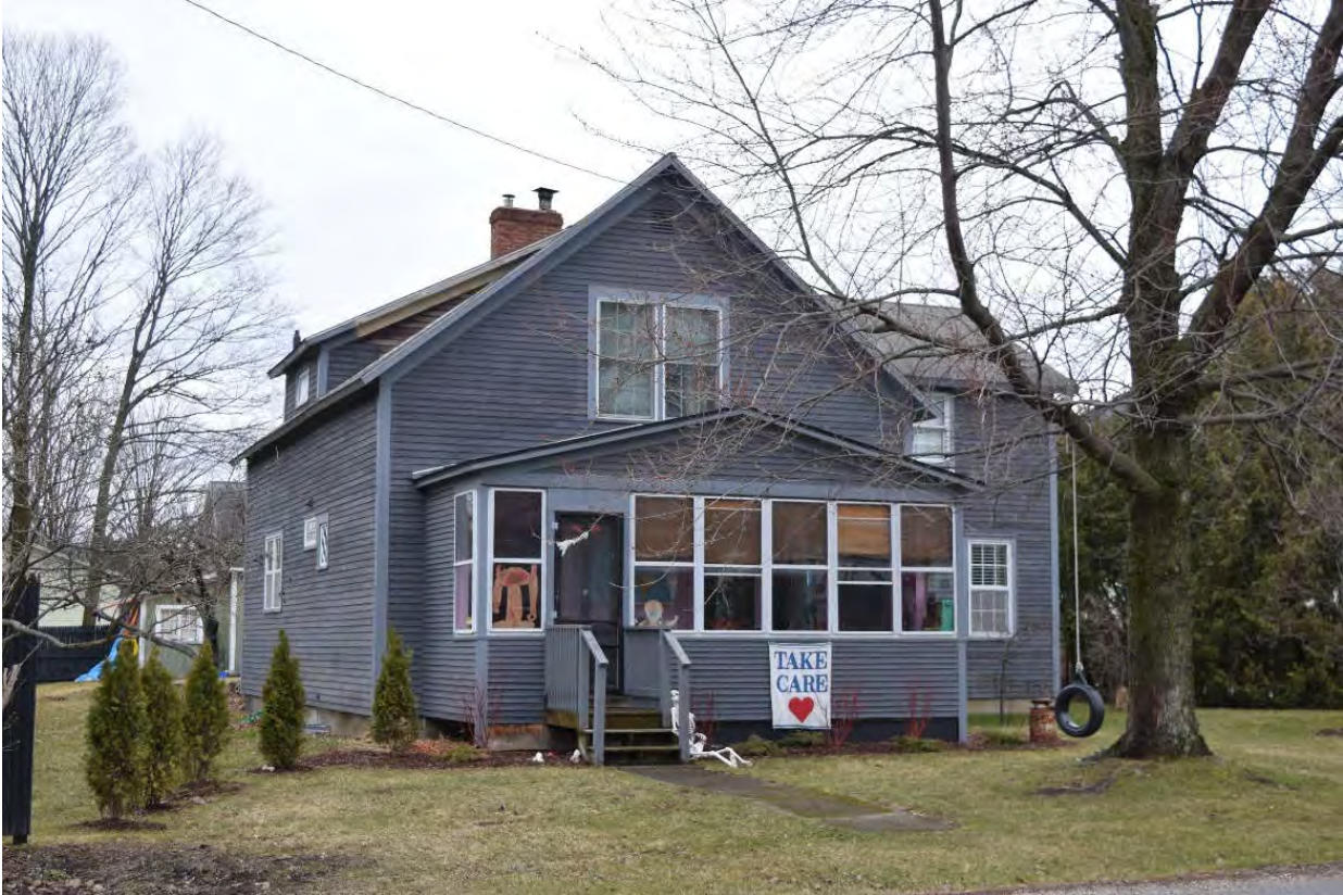
Photo 27. View of Structure 10 at 60 West Pleasant Street, looking north-northeast.
