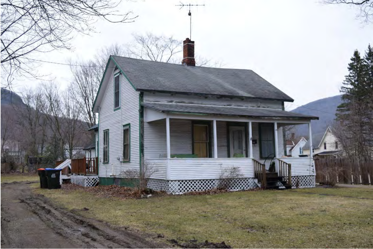
Photo 46. View of Structure 17 at 20 Munsill Avenue, looking southeast.
