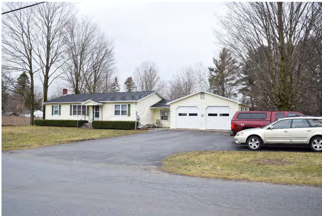
Photo 24. View of Structure 9 at 57 Munsill Avenue, looking west-southwest.
