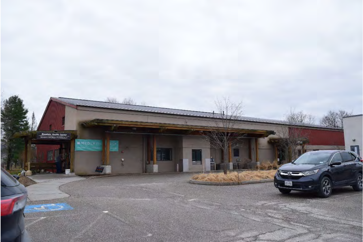
Photo 65. View of east building in the Structure 25 complex (61 Pine Street), looking south-southwest.
