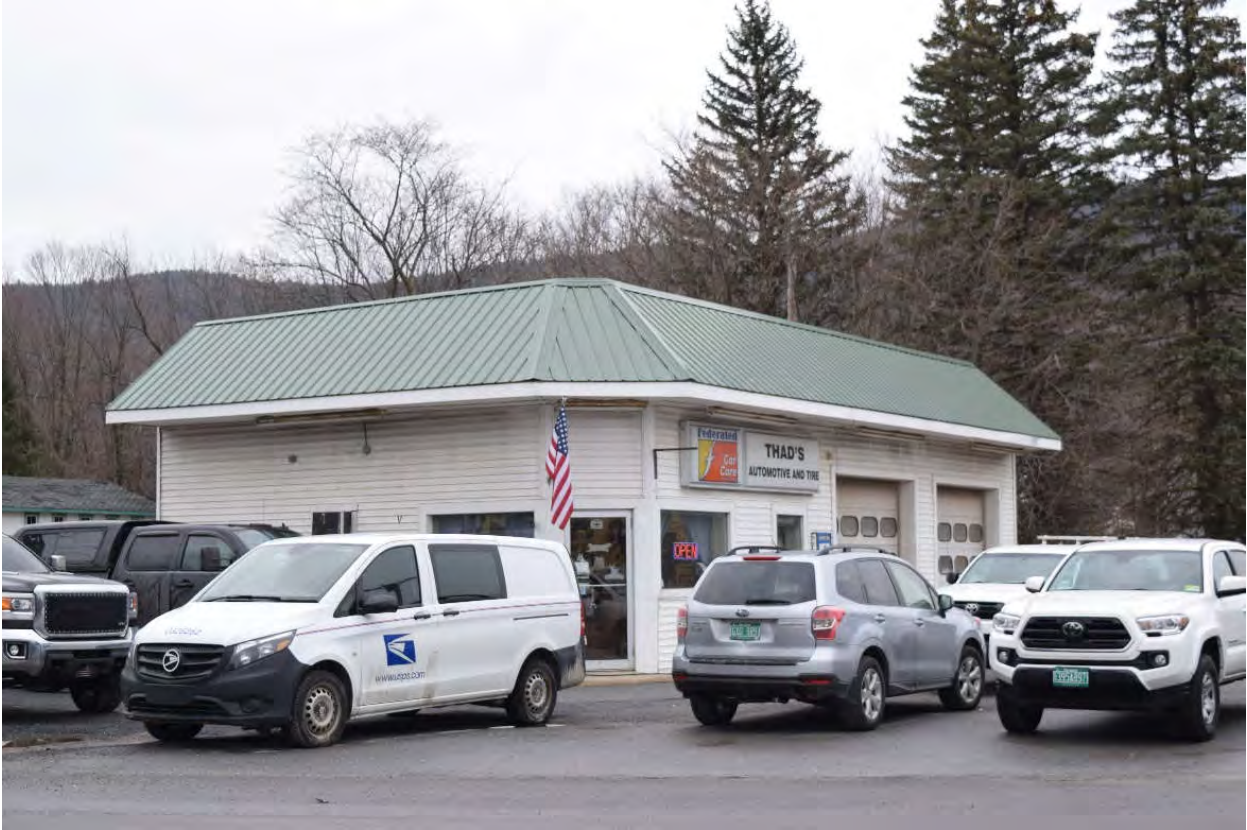
Photo 43. View of Structure 16 at 58 West Street, facing northeast.
