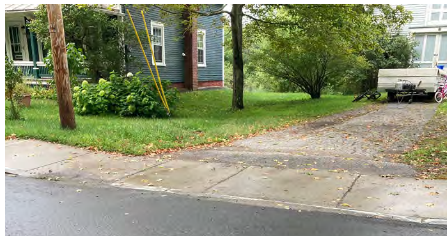
Typical Curbed Sidewalk at Driveway: A continuous concrete sidewalk surface, and curb, dips down to meet the existing driveway grade. See detail at right. While this configuration allows for a continuous surface, the "up and down" sidewalk travel can feel uneven, especially when driveways are close together.
