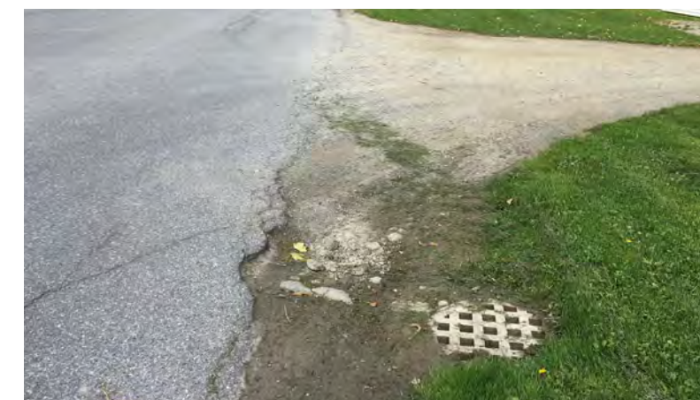
Move 3 Dry Wells
