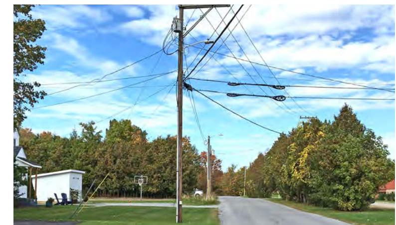
Move 4 Utility Poles
