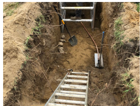
New Customer Service and Curb Stop
