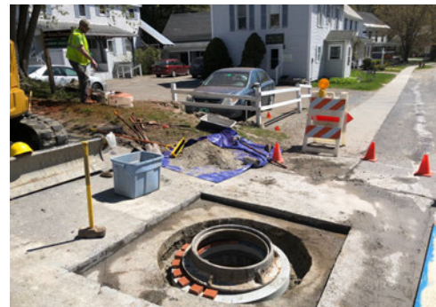
Manhole Rehab on East Street
