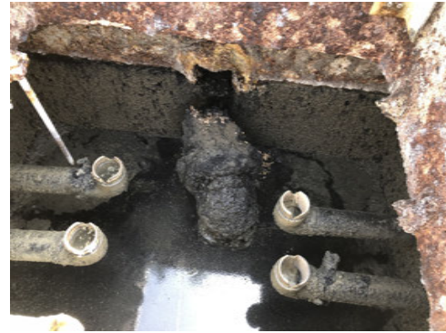
Sewer Splitter Box Rotten Inlet Pipe & Elbow
