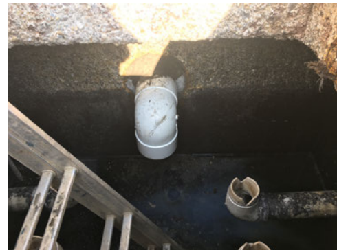
Sewer Splitter Box New Inlet Pipe & Elbow
