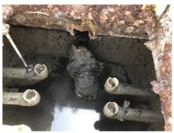
Sewer Splitter Box Rotten Inlet Pipe & Elbow
