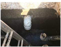
Sewer Splitter Box New Inlet Pipe & Elbow
