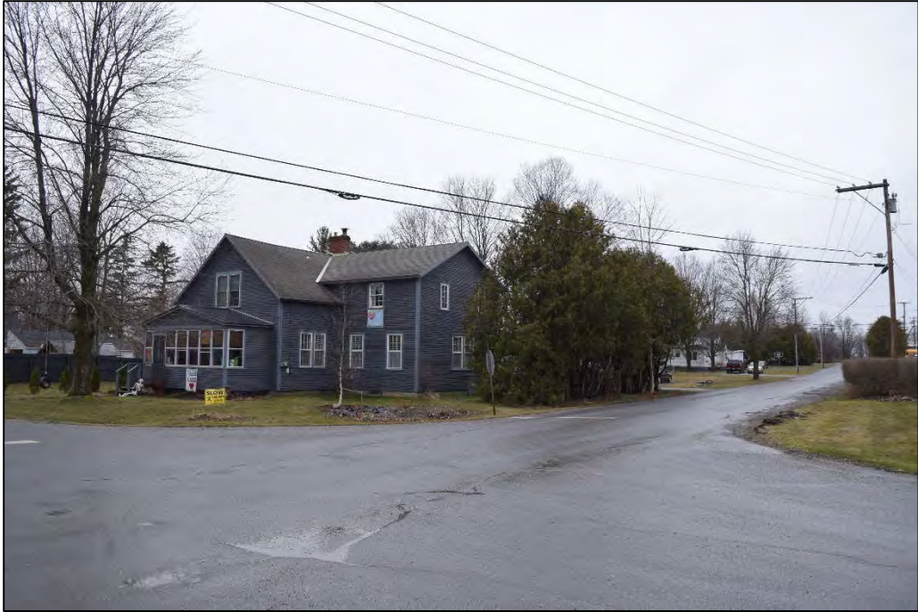
Photo 6. Intersection of Munsill Avenue and Pleasant Street. View to the northwest.
