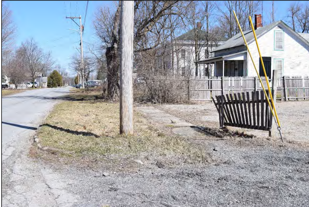
Photo 2. Remnant of sidewalk along the east side of the APE. View to the north.
