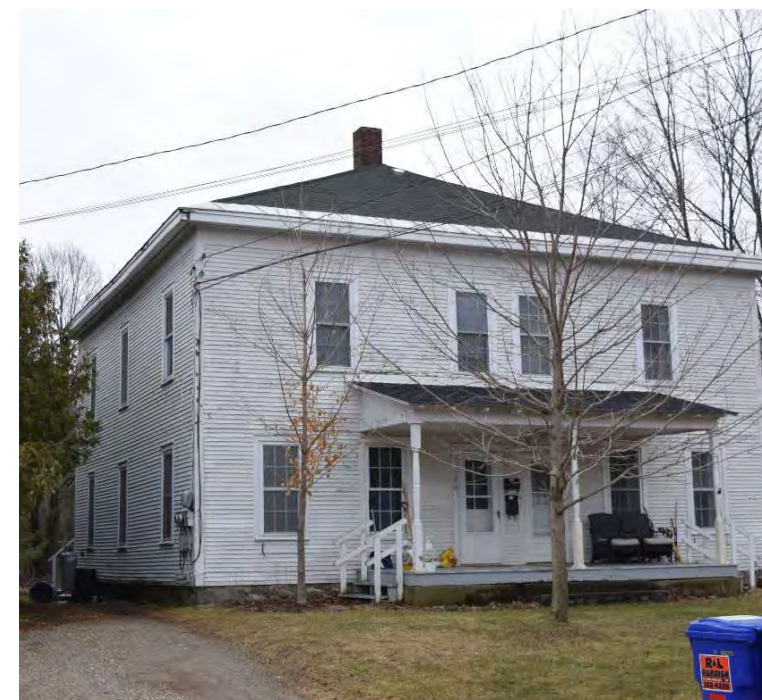
Two views of 28-30 Munsill Avenue. Per the HRI, this property retains sufficient historic integrity to be listed on the National Register of Historic Places. However, as it may relate to potential adverse impacts of sidewalk construction along this property frontage, note the presence of only young trees in the front yard of this building.
