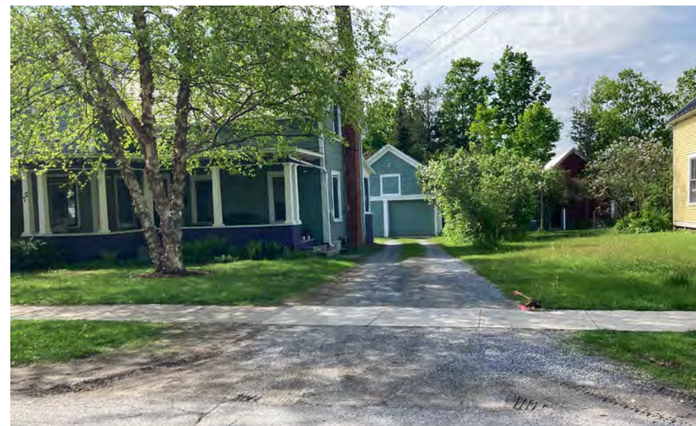
Typical Buffered Sidewalk at Driveway: A continuous and level-flush concrete sidewalk continues across the driveway surface.
