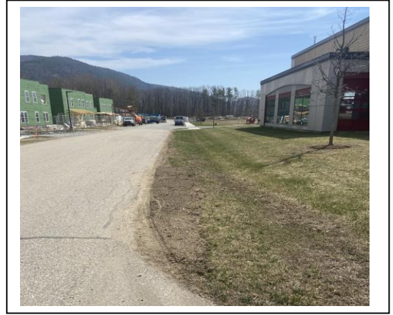
Recently repaired grass areas along driveway
