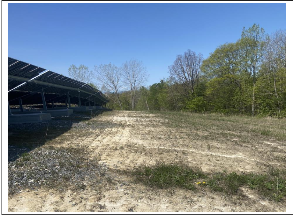
Photo #3 – Area in Need of Vegetative Cover
