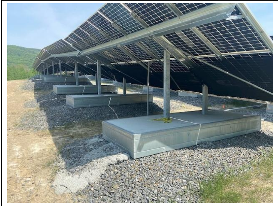
Photo #5 – Solar Array Foundation
