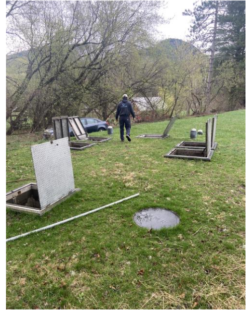
Septic tank access hatches
