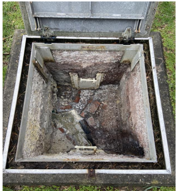
Septic tank outlet trough
