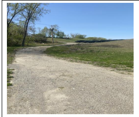
Lower Driveway Entrance
