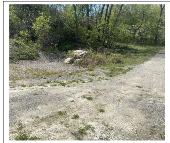
Grading at Stormwater Infiltration Basin
