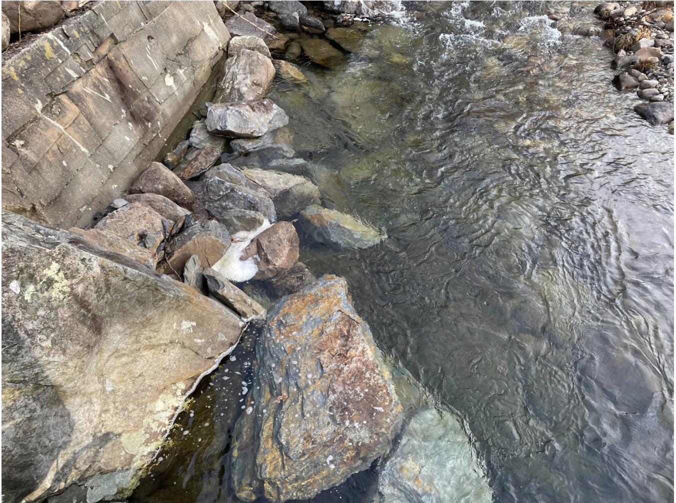
Figure 1: Installed stone at based of large boulder.
