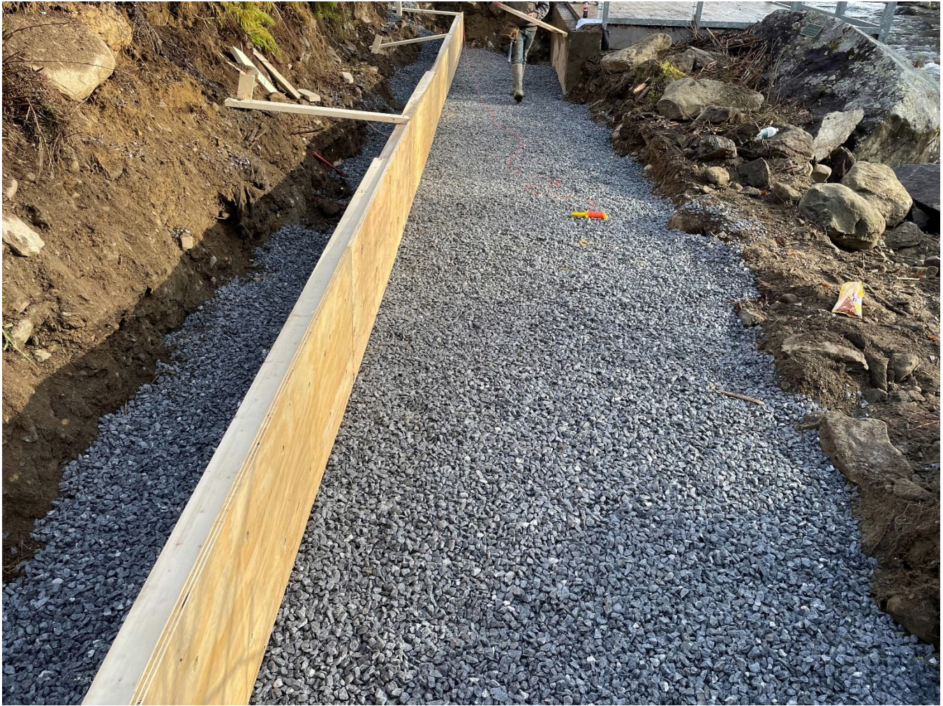
Figure 2: Prepared base for walkway installation and start of concrete forms.
