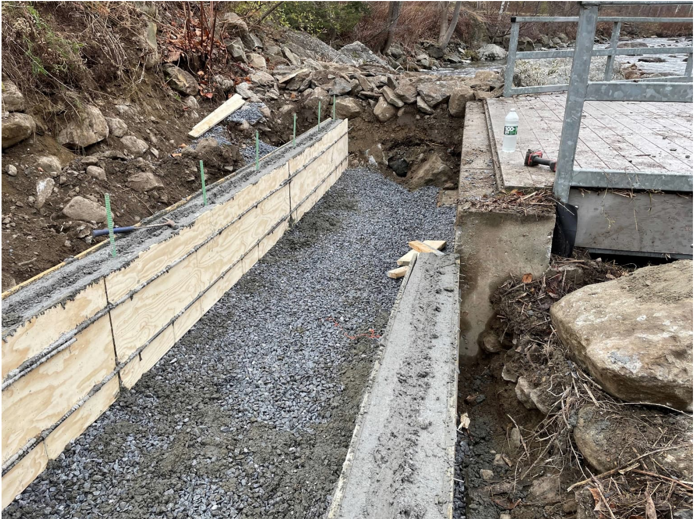
Figure 2: Curing walls looking down the path towards the platform.
