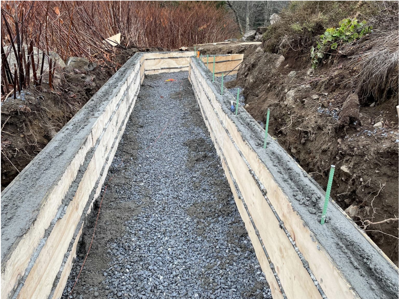
Figure 1: Curing walls looking up the path from the platform.
