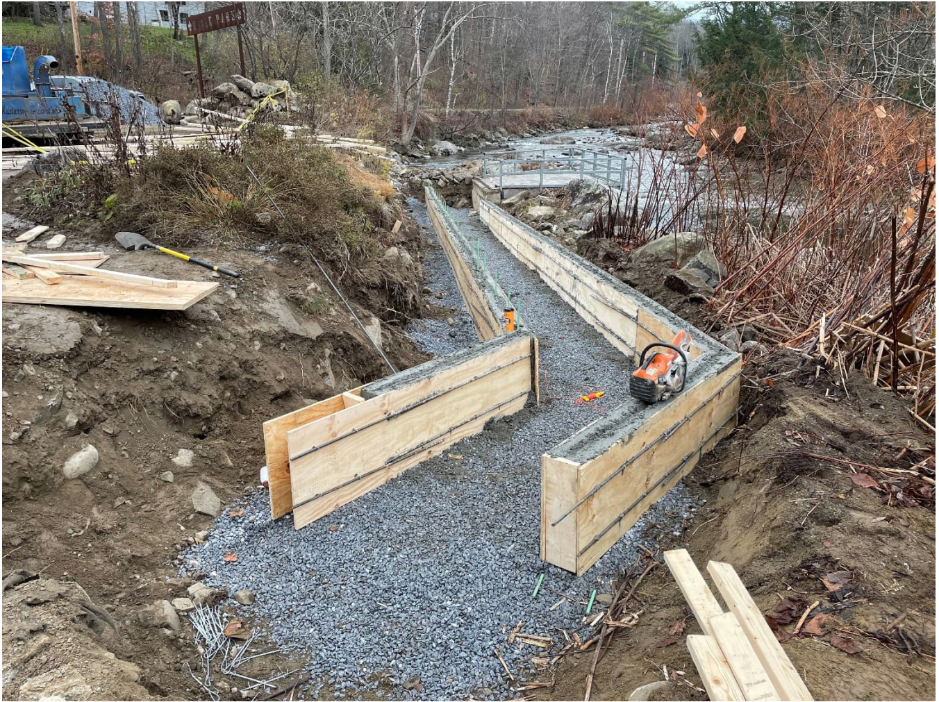
Figure 3: Curing walls looking down the path towards the platform.
