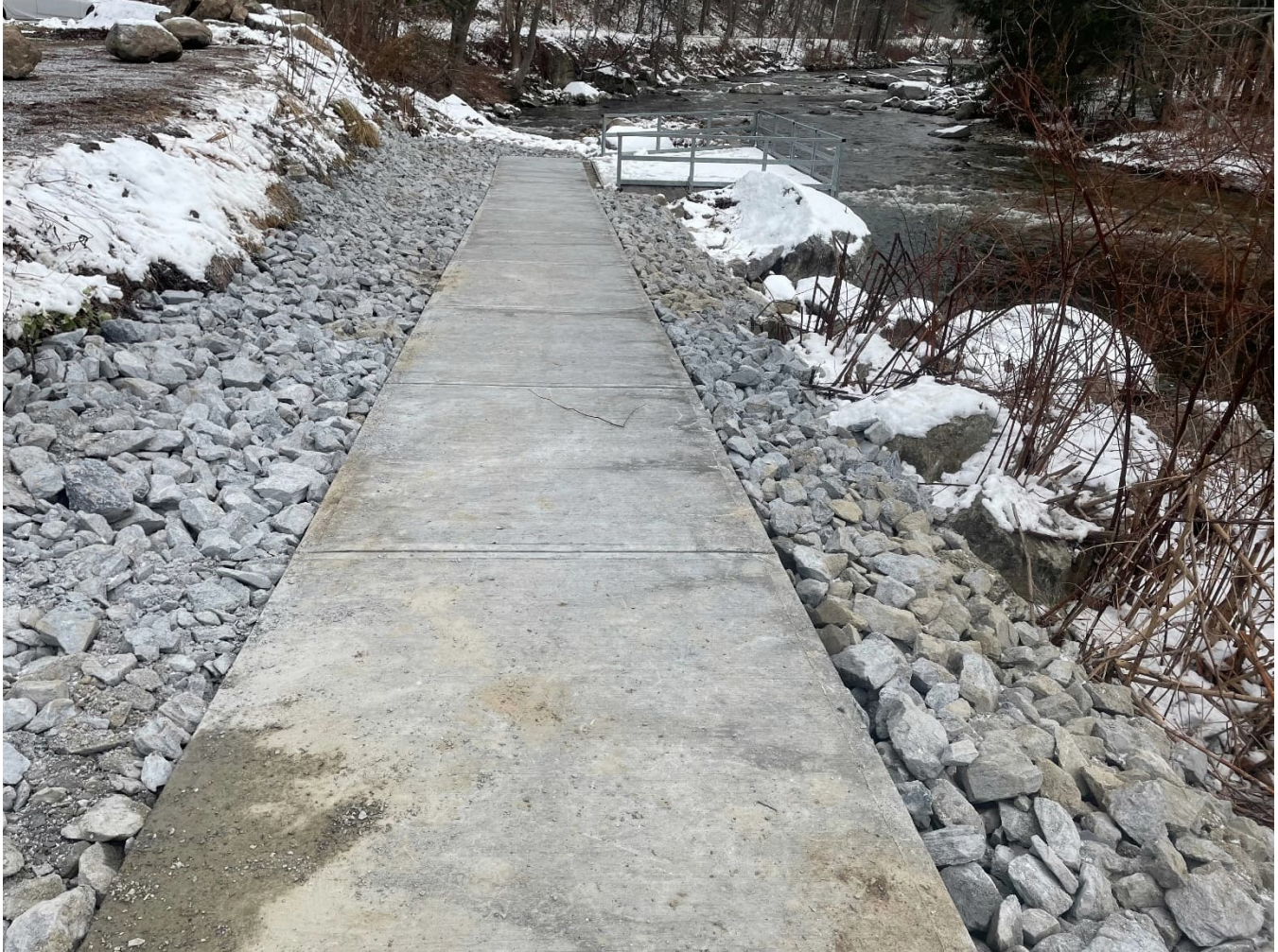
Figure 1: Completed concrete walkway looking upstream towards platform.
