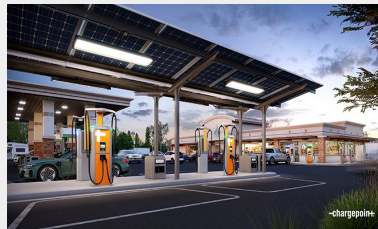
Electric vehicle charging stations
