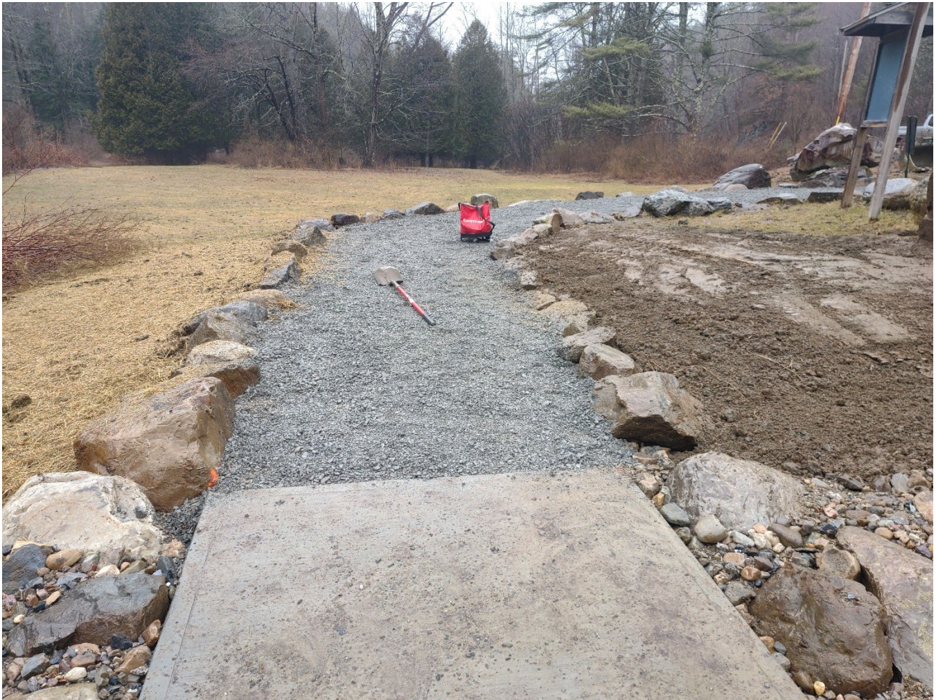
Figure 6: Restored gravel path lined with small boulders, restoration of lawn area underway to the right of the path in photo.
