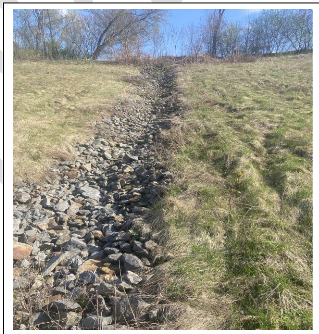
Photo #4 – Typical Drainage Swale
