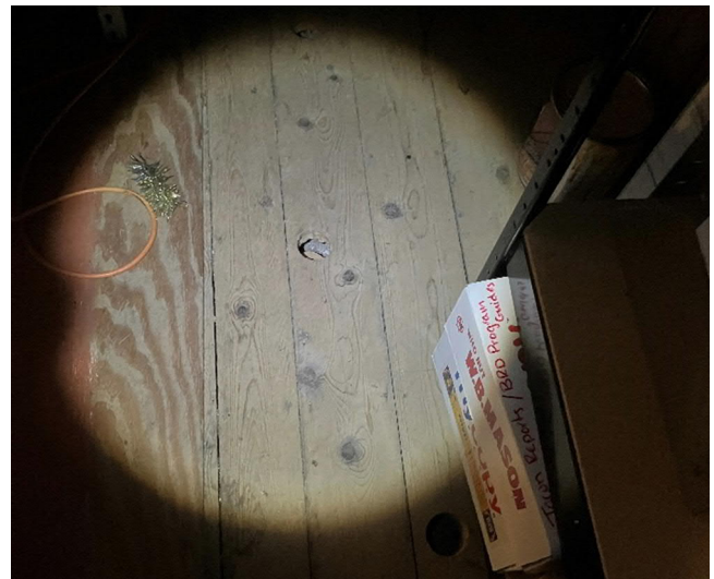
Figure 24 – But up close not much insulation is in the floor
