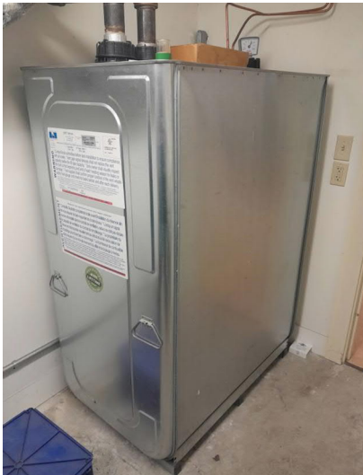
Figure 2 – Existing Oil Storage Tank
