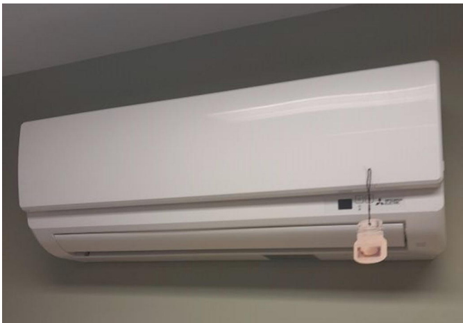
Figure 48 – Existing Interior Heat Pump Ductless Units
