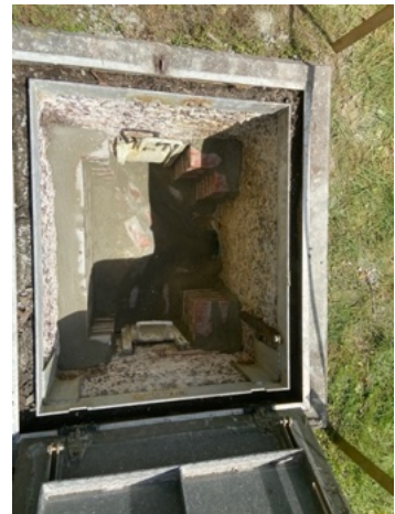
Rehabilitated Effluent Sewer System post-rehabilitation
