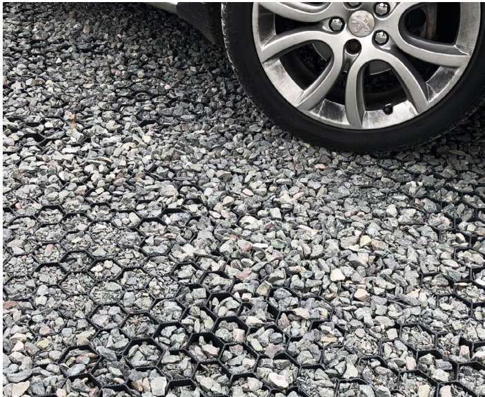
Proposed stabilized aggregate surface of accessible parking spaces
